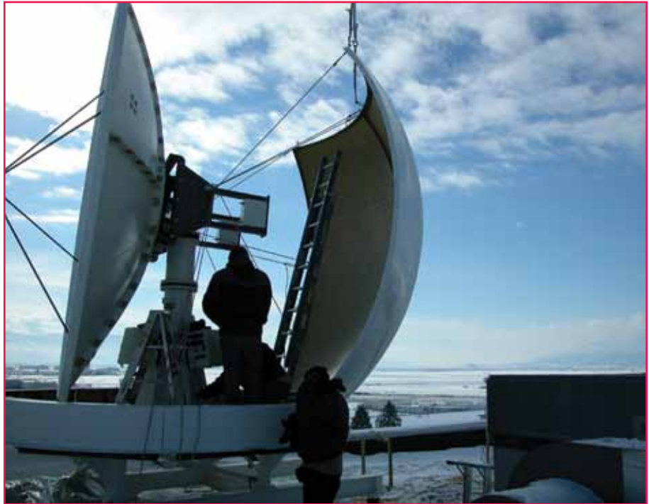
A satellite receiving dish installed on the roof of the fire lab collects infrared data several times a day to map “hot spots” across the United States. Photo: Forest Service.
