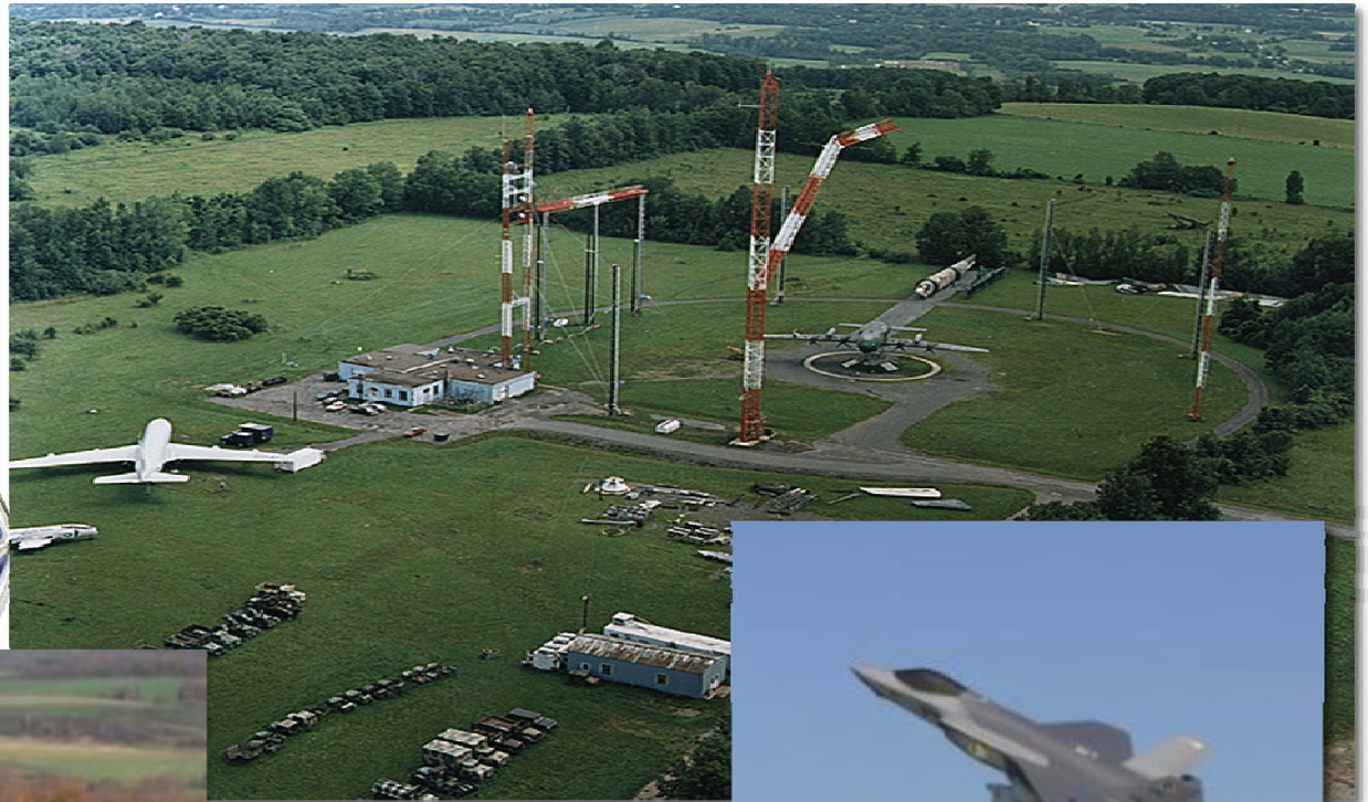
Stockbridge Test Facility
