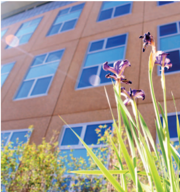
The RSF serves as a blueprint for achieving ultra-energy efficiency and net-zero energy performance. Photo by Heather Lammers, NREL/PIX 17515
