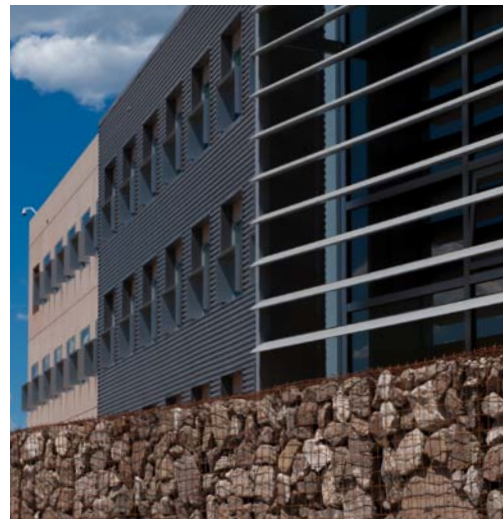
Gabion walls. Photo from Frank Ooms Photography
