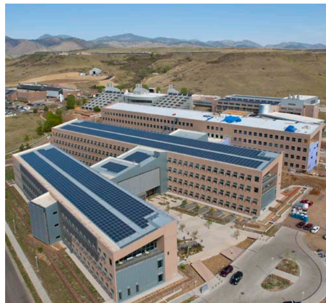
The RSF includes 450kW of roof-mounted PV panels. Photo by Dennis Schroeder, NREL/PIX19089
