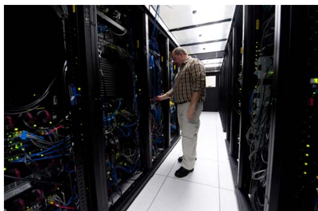
The RSF data center features an extremely low power usage effectiveness ratio of 1.13. Photo by Dennis Schroeder, NREL/PIX 18780
