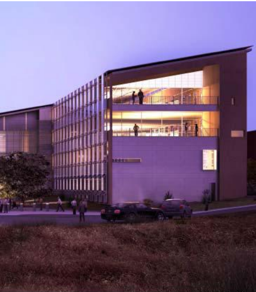
View looking East into the Entry Plaza
