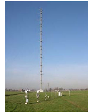
The 213m tower at the Cabauw meteorological site in The Netherlands. More information can be found online at http://www.cesar-observatory.nl .
