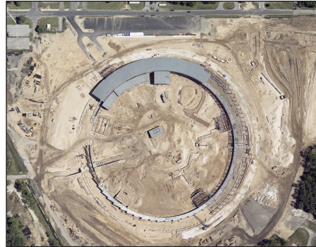
Viewed from above during construction in 2010, NSLS-II will be complete in 2015
