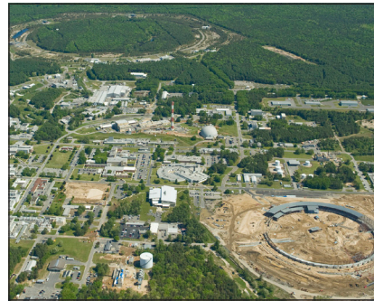
Brookhaven Lab's major facilities include the Relativistic Heavy Ion Collider (top) and future National Synchrotron Light Source II (bottom).
