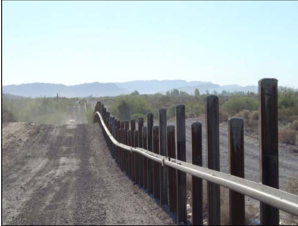
Figure 1-2. Post-on-Rail-Style Vehicle Fence (Fence Type VF-1)
