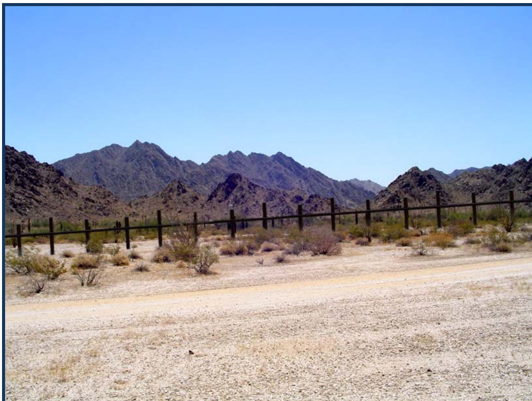
Figure 3-4. Photograph of Fencing and Cabeza Prieta Mountains
