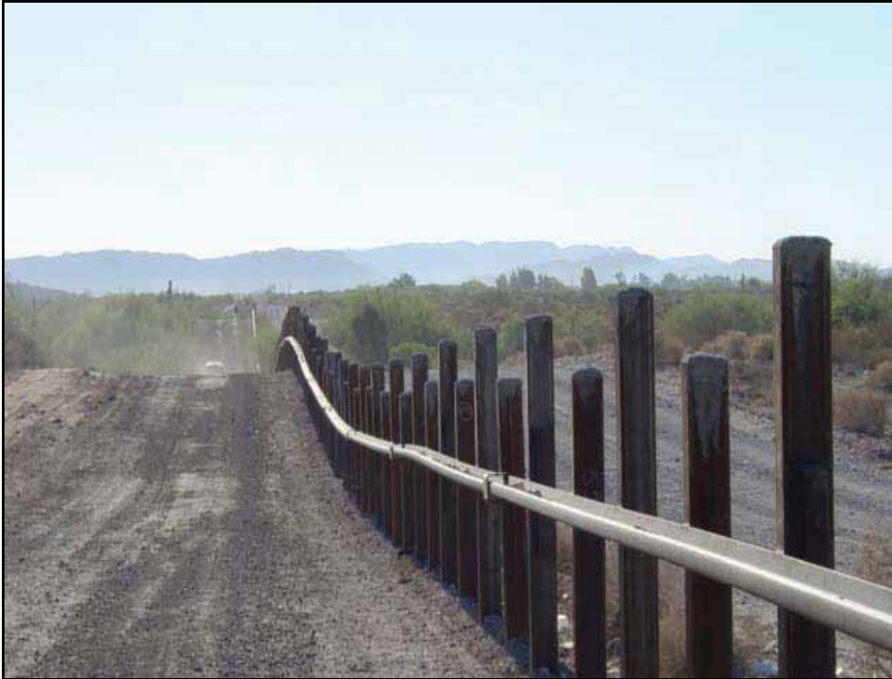
Figure B-1. Post-and-Rail Vehicle Fence (VF-1)
