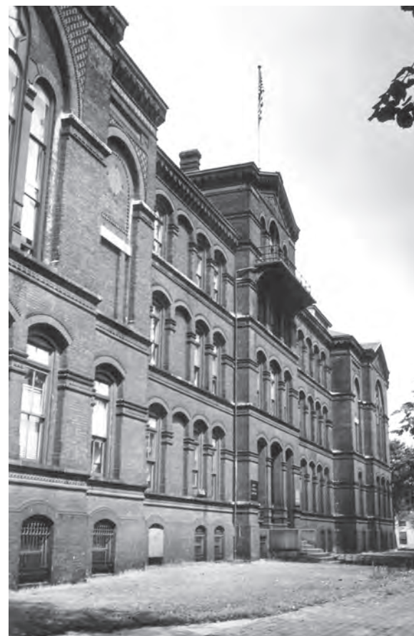
Adolf Cluss’s 1885 design for the Army Medical Museum, located on the Mall’s south side at 7th Street, SW, was built by Colonel Thomas Lincoln Casey using inexpensive brick, terra cotta, and iron materials. The building, on the site now occupied by the Hirshhorn Museum, was razed in 1969. (Photographed ca. 1940s)
