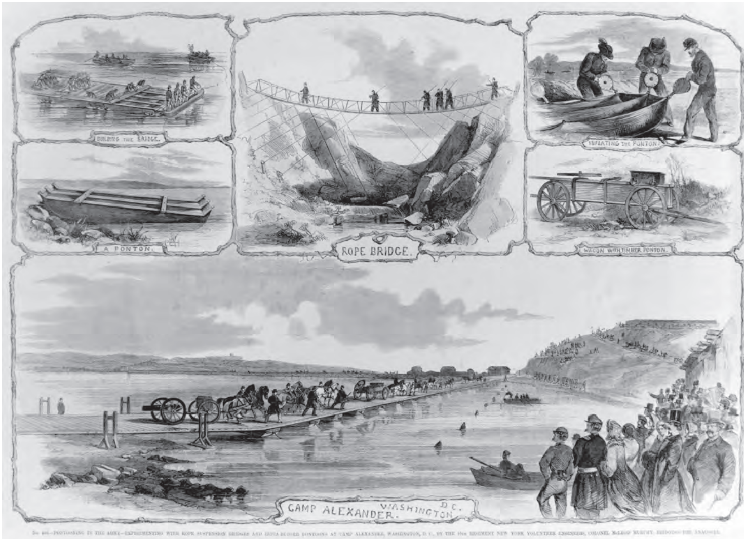
Lithograph of the 15th New York Volunteer Engineers experimenting with rope suspension bridges and India rubber pontoons and ponton bridges at Camp Alexander on the Anacostia River during the Civil War Office of History, Corps of Engineers
