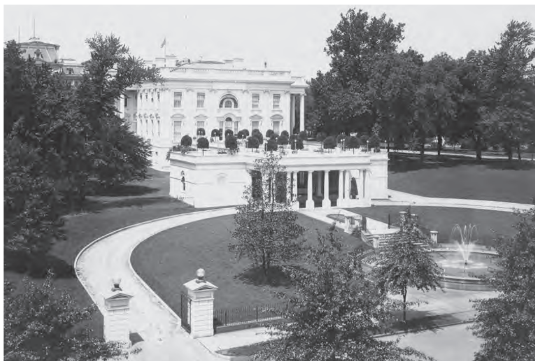
New White House east entrance and terrace, 1903
