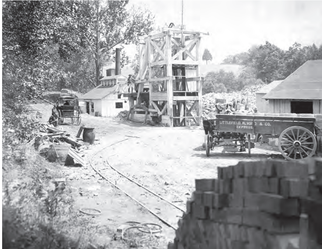
Foundry Branch shaft leading to the tunnel connecting the distributing reservoir and the new reservoir, 1884. The engineers built three shafts at Foundry Branch, Rock Creek, and Champlain Avenue. Washington Aqueduct Division, Baltimore Engineer District
