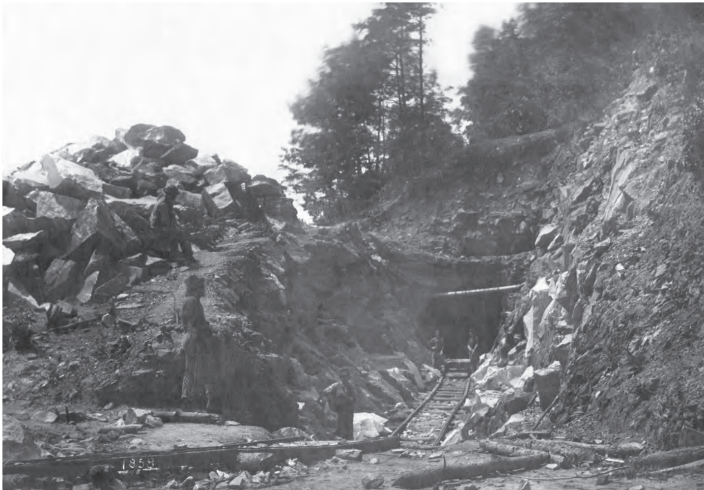
Digging tunnels for the Aqueduct, August 1858 National Archives no. 77-HCS-1B4
