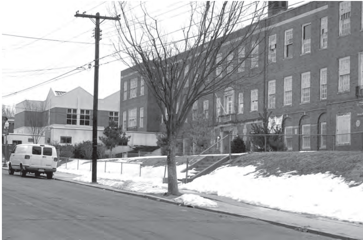
Following completion of a new building for Barnard Elementary School on 4th Street, NW, between Crittenden and Decatur Streets, the 1926 structure was demolished to make room for playgrounds. Baltimore Engineer District
