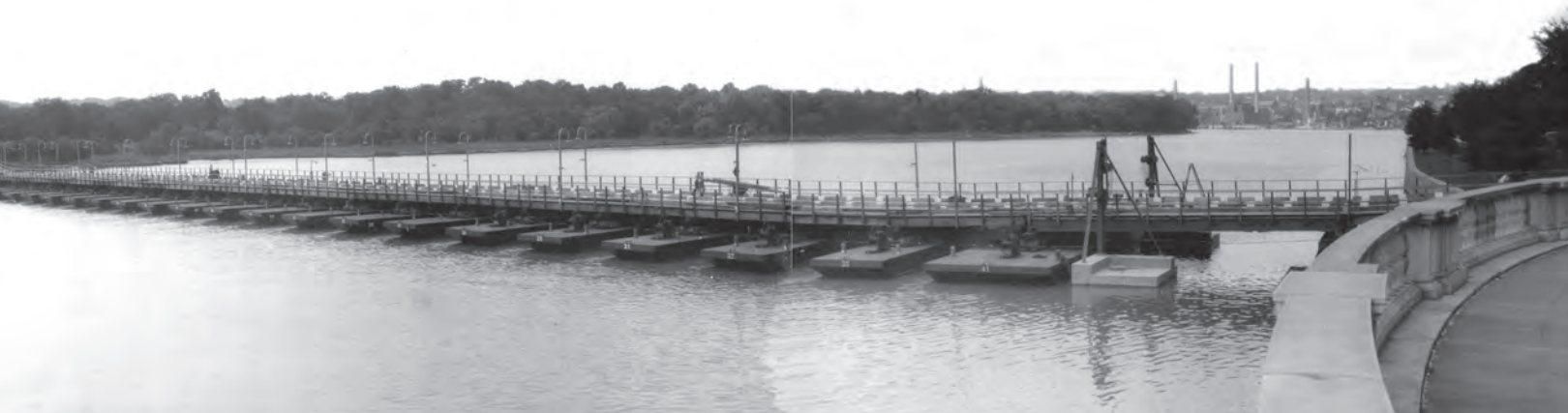
(Top) Emergency Railroad Bridge, August 1942. The Washington Engineer District built this additional, temporary crossing over the Potomac River from Shepherds Landing, D.C., to Alexandria, Virginia, to transport goods and troops in a national emergency. Authorities worried that the bridge immediately to the north was the only rail crossing of the southern Potomac River. National Archives no. 77-RH-141B-1
