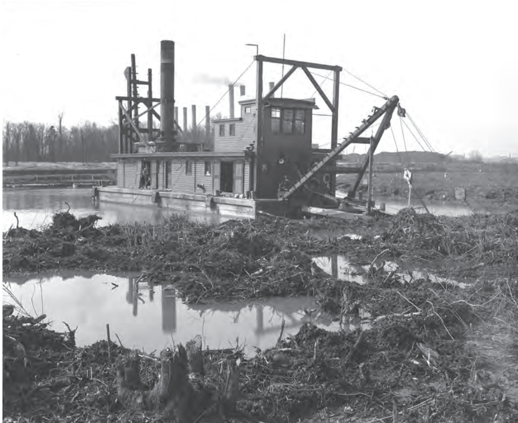
The Corps of Engineers' dredge Dalecarlia at work on Anacostia River reclamation (n.d.). Like the reclamation of the Potomac flats, the Anacostia work required extensive dredge and fill operations to drain and reclaim its extensive marshland. Office of History, Corps of Engineers
