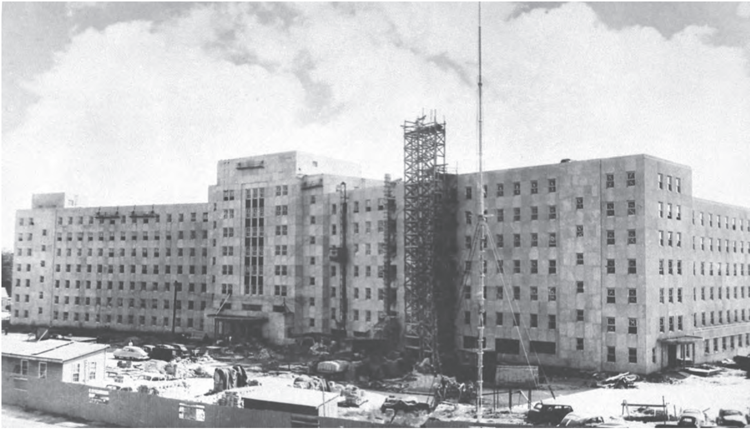
The 850-bed residence hall under construction at the U.S. Soldiers' Home, 1952, was named for Winfield Scott, who was instrumental in the establishment of the Soldiers' Home in 1851. Office of History, Corps of Engineers
