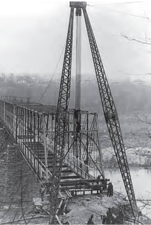
Chain Bridge undergoing repairs, 1928. One end of the wrought-iron bridge built by Babcock in 1874 was lifted to repair one of its piers.
