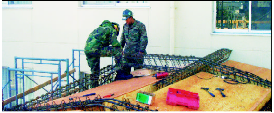
Photos courtesy of Seabees
