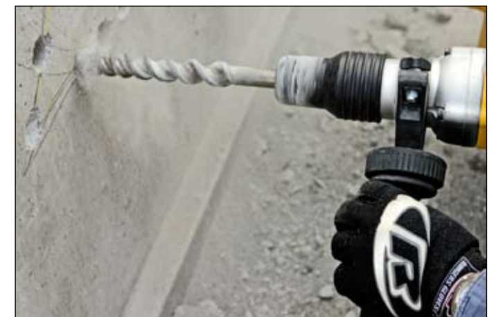
A station firefighter drills another hole into concrete in preparation to make a clean breach into an enclosed area where a victim is trapped during a final exercise in urban search and rescue training here Sept. 25. The purpose of a clean breach, as opposed to a dirty breach, is to prevent as much rubble and debris as possible from falling in and further injuring the victim. Photo by Lance Cpl. Joseph Marianelli
