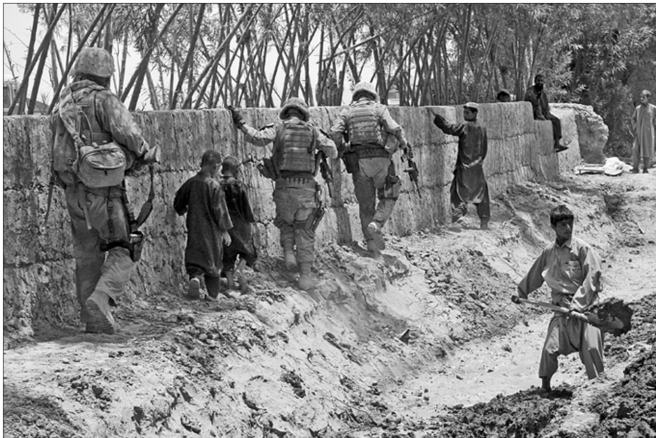
HELMAND PROVINCE, Afghanistan — Marines with the 24th Marine Expeditionary Unit help Garmsir citizens make bricks to rebuild their homes. The MEU has focused efforts on Garmsir's infrastructure since kinetic operations slowed in June. Cpl. Randall Clinton
