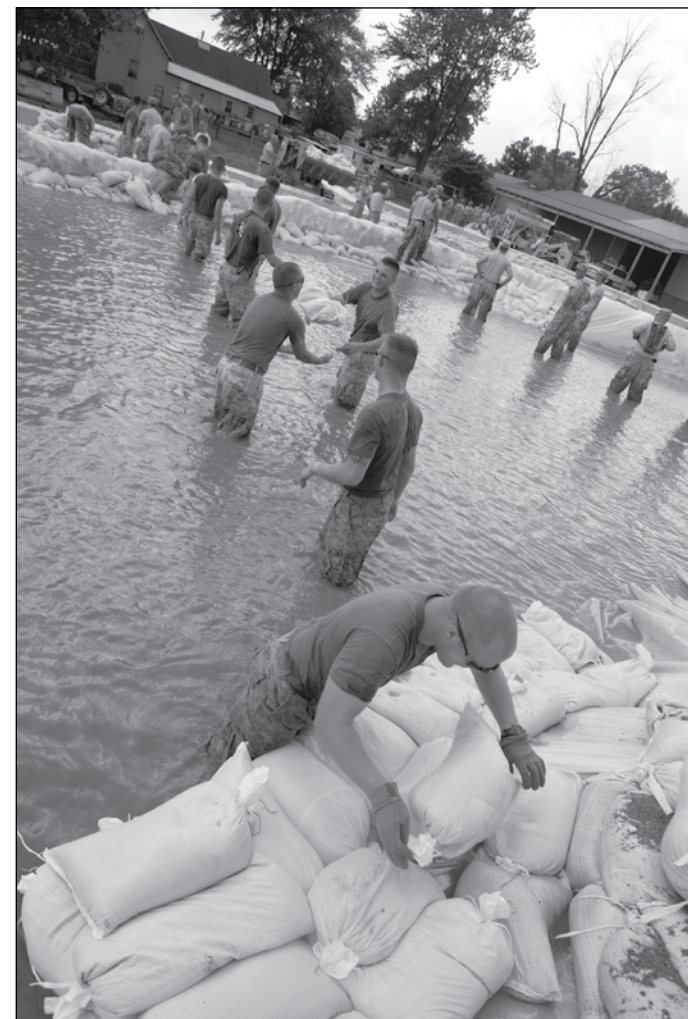
Marines and sailors of 26th Marine Expeditionary Unit stack sand bags to reinforce the levees June 9 in Elnora, Ind. Local authorities in Elnora requested the 26th MEU to provide support to reinforce the levees from flooding of the White River.
