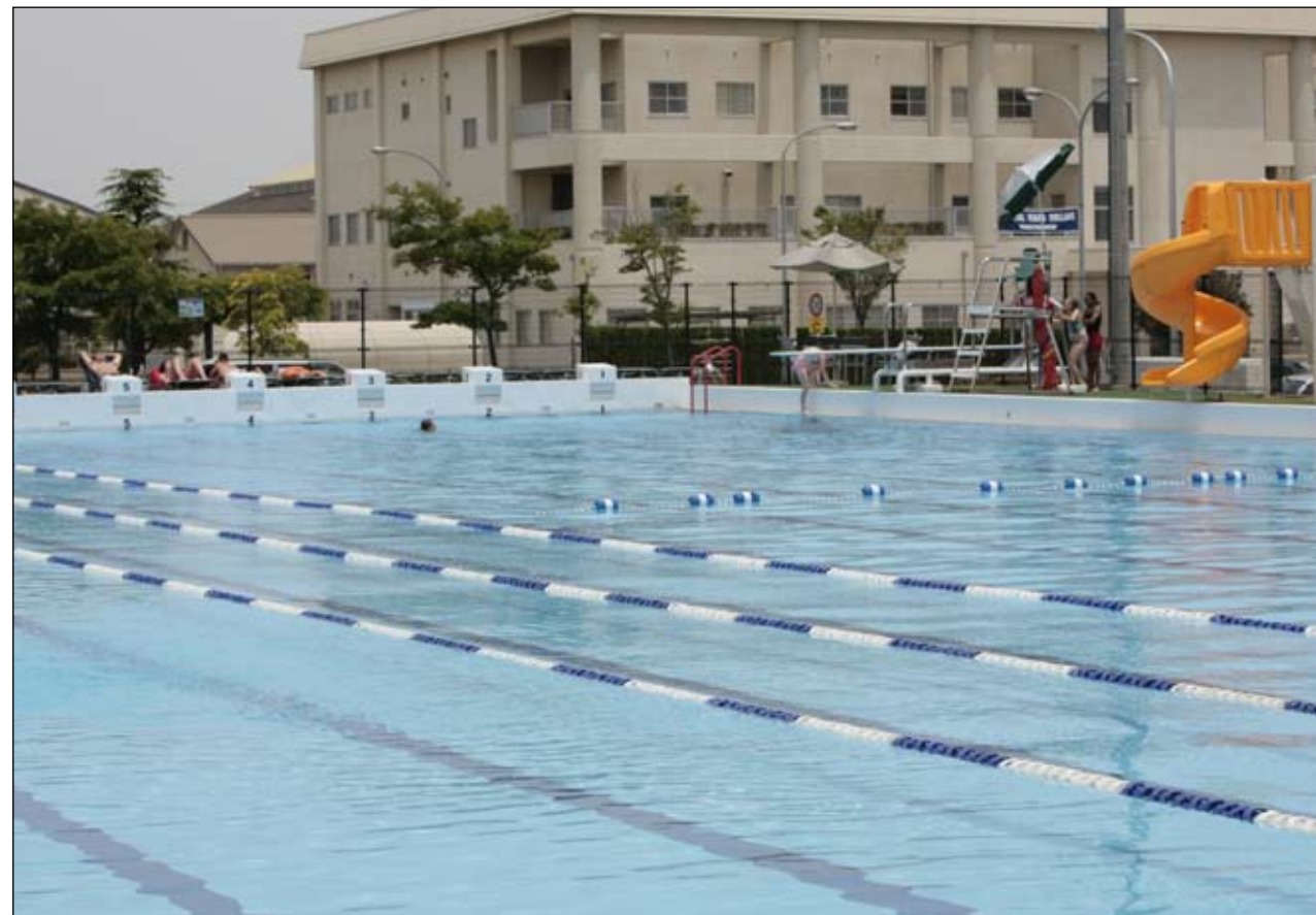
The pool is split into five parts. One for swimming laps, another for the shallow end, two for the slide areas and the children's area.
