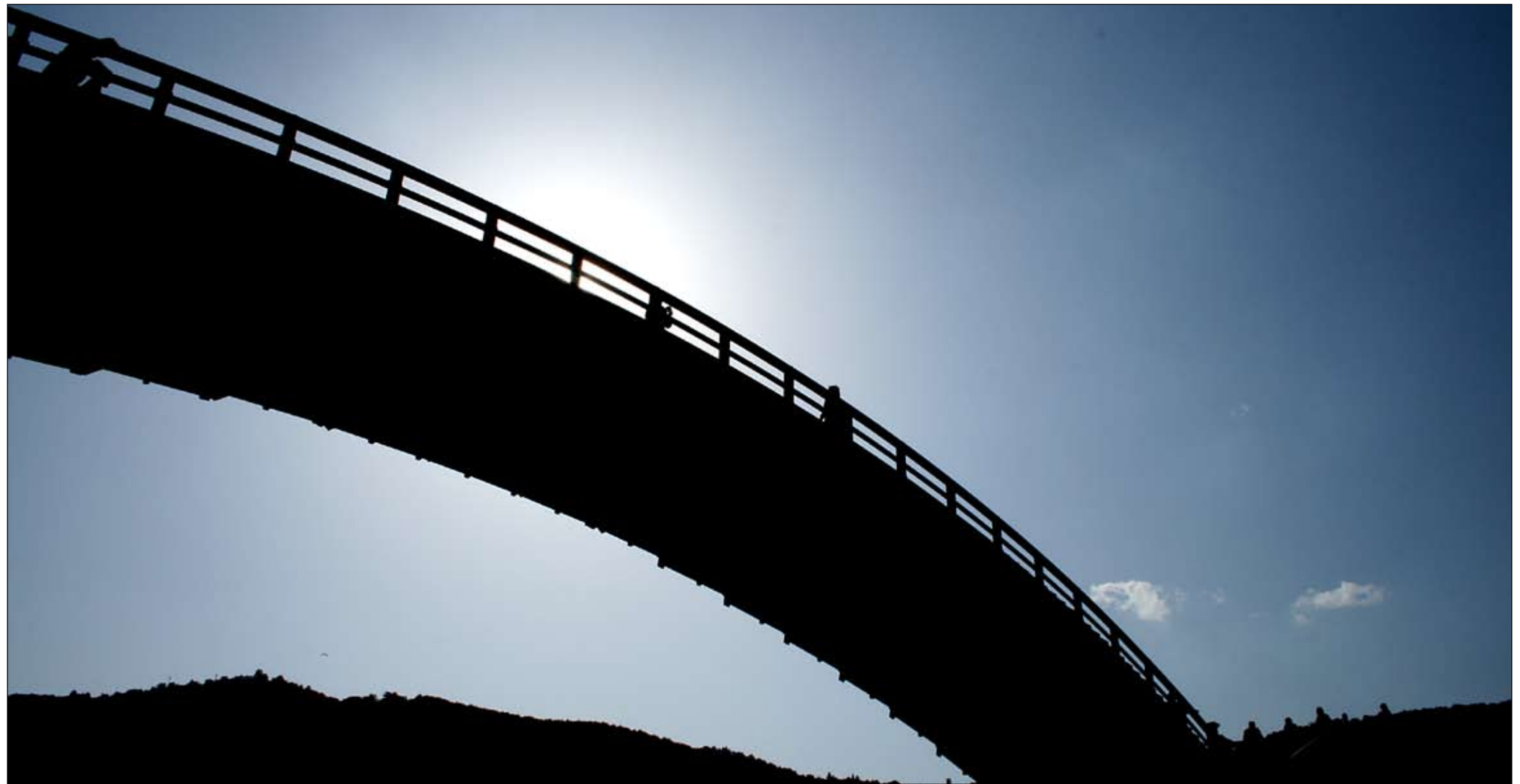
Iwakuni's Kintai Bridge and its area scenery attracted thousands of visitors April 4. The monumental cherry blossoms were in full bloom along the banks of the Nishiki River. Photo by Cpl. Josh Cox
