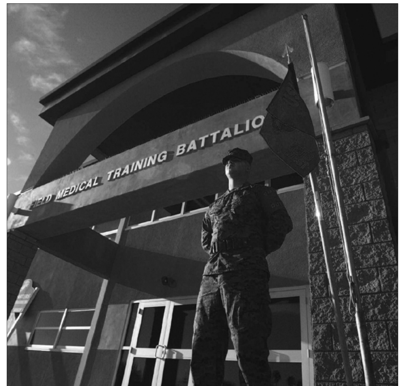
Petty Officer 3rd Class Randall Winters, Field Medical Training Battalion, Training Education Command, stands duty at the newly renovated FMTB facility, which received its first overhaul in 50 years. The upgrade cost more than $4 million and included state-of-the-art equipment to enhance the curriculum. Photos by Sgt. Michael T. Knight
