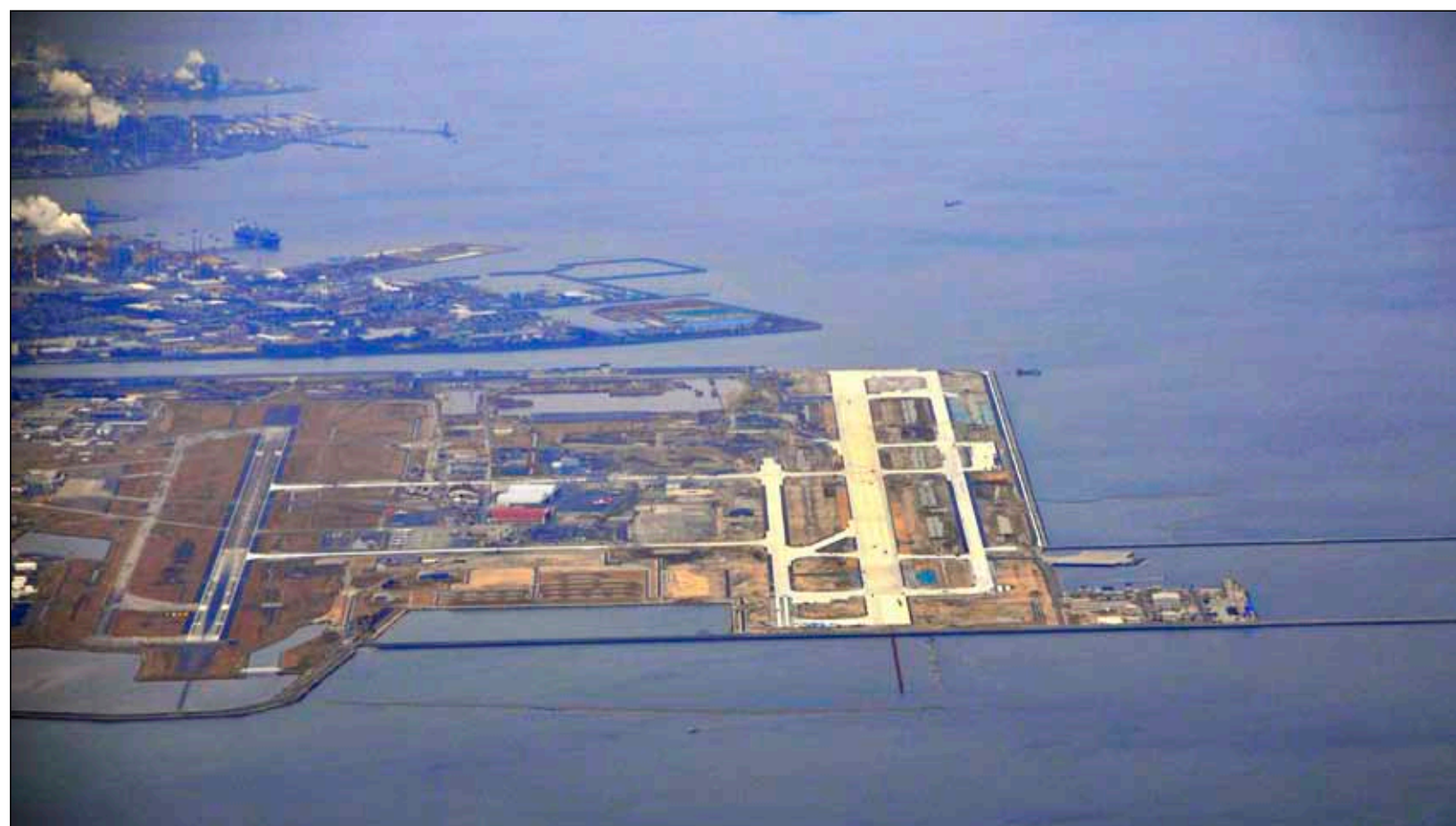
PHOTO COURTESY OF THE CHUGOKU-SHIKOKU DEFENSE BUREAU An aerial view of the fully constructed runway. A commissioning ceremony was held at the runway here to officially open it to flight operations May 29. The historic ceremony marked the conclusion of the $2.6 billion, 13-year construction effort.
