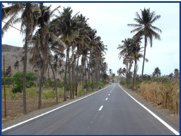
Now, the new road between Órgãos and Pedra Badejo is 10 kilometers long and 6 meters wide, has a drainage system, signage, lighting, and all safety and environmental standards in place. Nearly 12,500 people are expected to benefit from this road now, increasing to more than 15,000 over the next twenty years.
