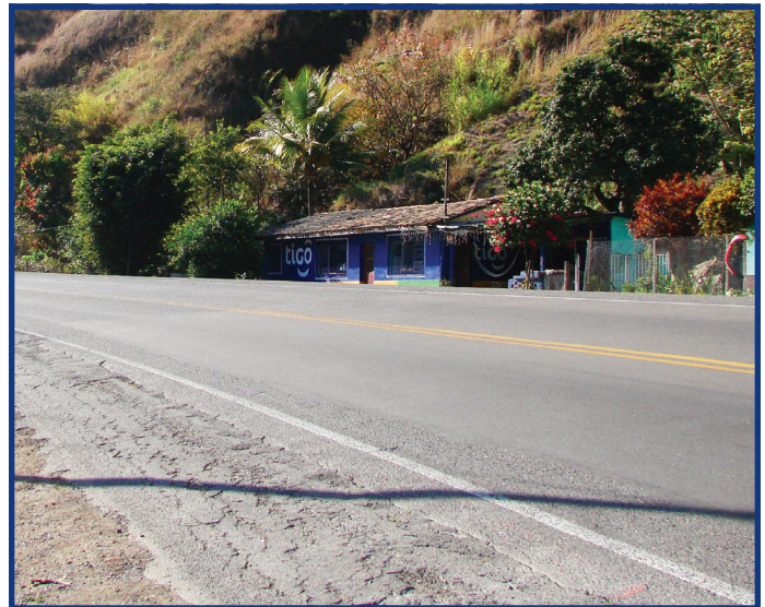
A segment of Highway CA-5 North.
