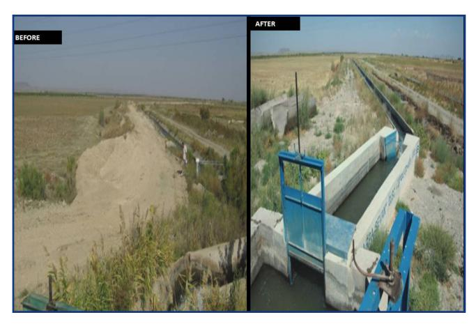
In place of broken concrete, Armenia's irrigation canals are now equipped with well-designed structures that maintain desirable water levels both upstream and downstream at all times during the growing season.
