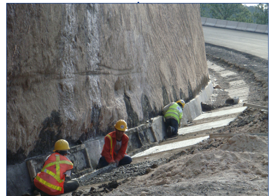
Road construction and rehabilitations have employed over 4,000 people.
