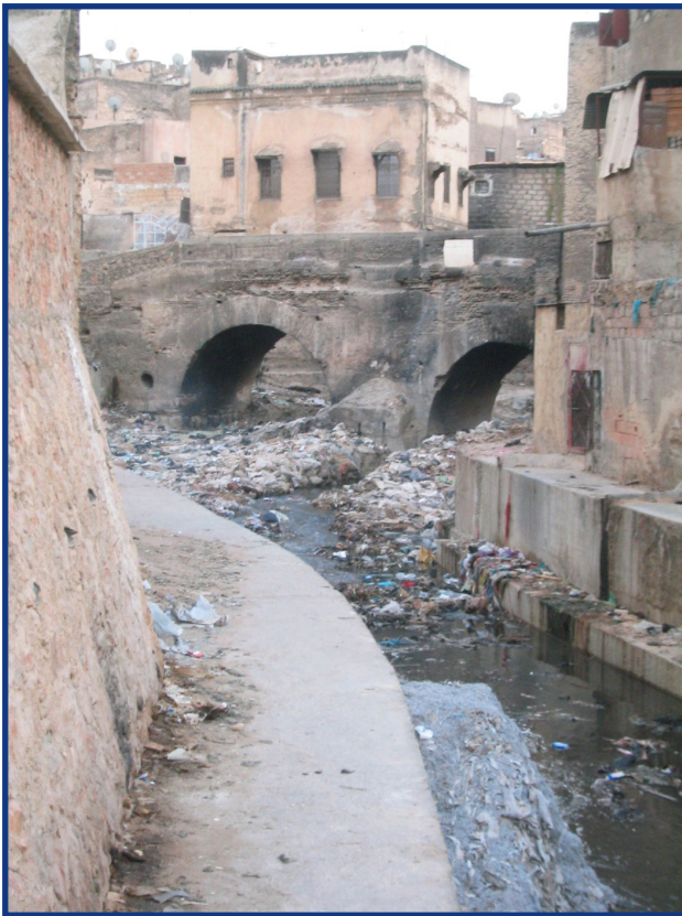
Existing conditions at the Bim Lamdoun Bridge
