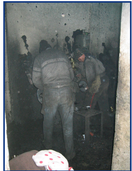
Metal workers work in cramped quarters in PLY.
