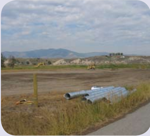
Constructed wetland cell after initial vegetation removal and shaping.
