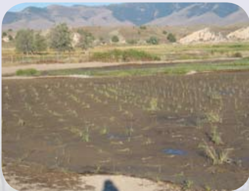
Constructed wetland cell after planting and initial flooding cycle.
