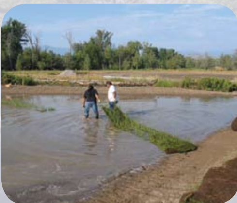
Placement of pre-vegetated mats within a constructed wetland cell.
