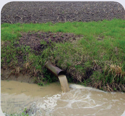
Tile drainage—the major pathway for nitrate export from cropland in Honey Creek. Photo by Hans Gottgens
