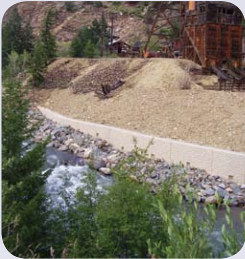
The old Maud Monroe mine will be remediated and preserved as a historic mining tourism center.
