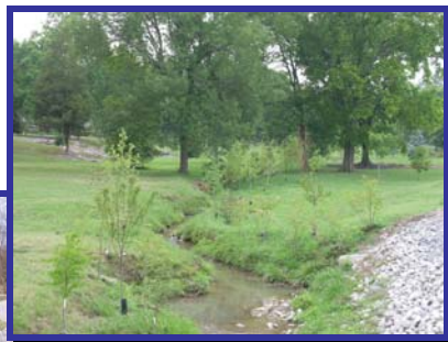
After restoration, the stream has riparian plantings, which will minimize pollutants, provide habitat and control temperature.
