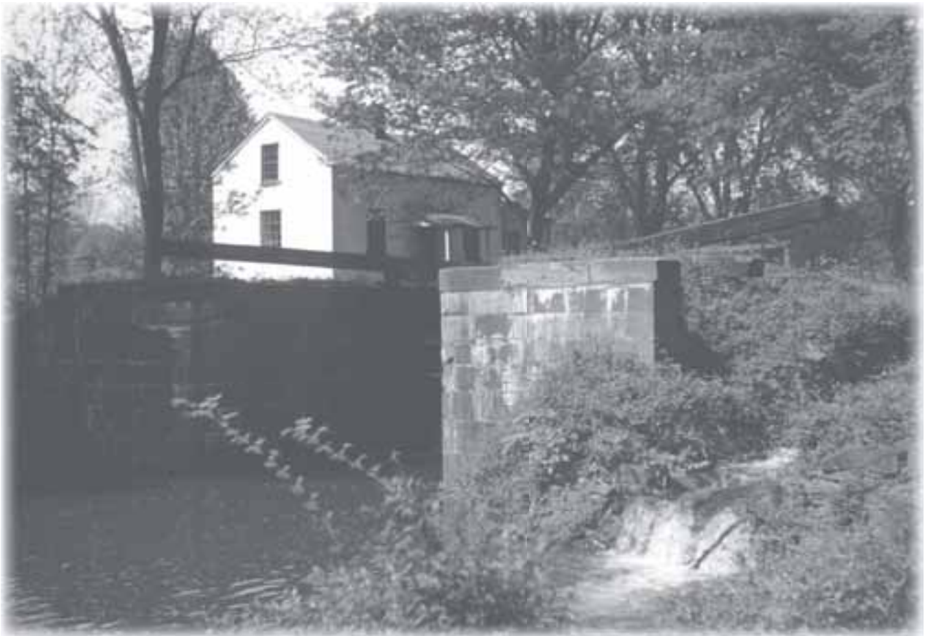
Lock 11 and lock house
