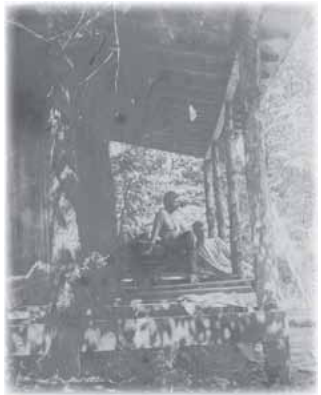
Wilfred Osgood and William Palmer building the porch, 1901
