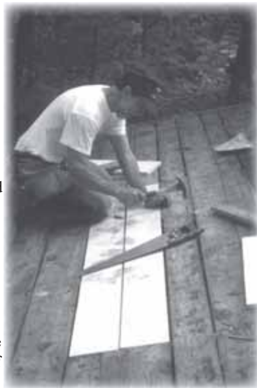
Repairs to the roof were made by a contractor
