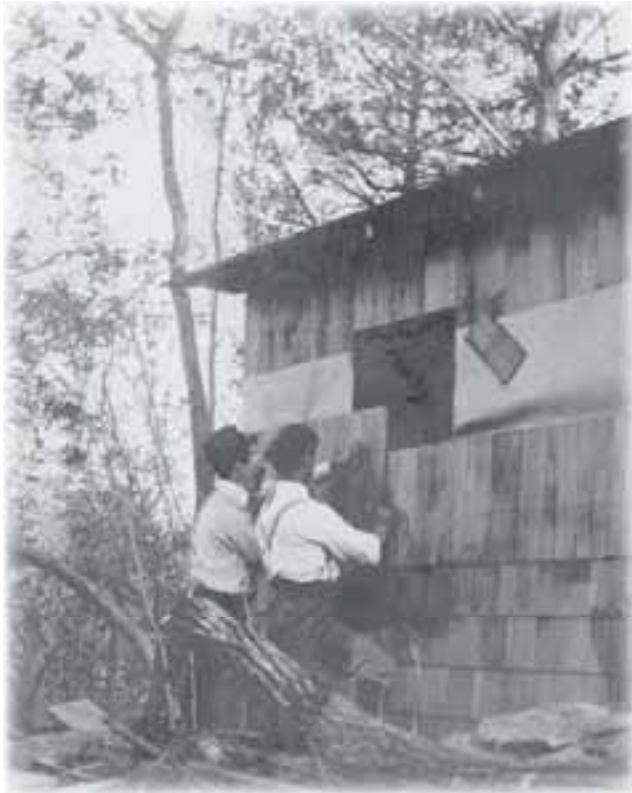
William Maxon and Edgar Brown installing shingles, 1901
