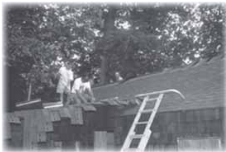
Members and friends volunteered to install new shingles
