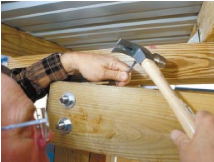
This is NOT the way this claw hammer was designed to be used.
