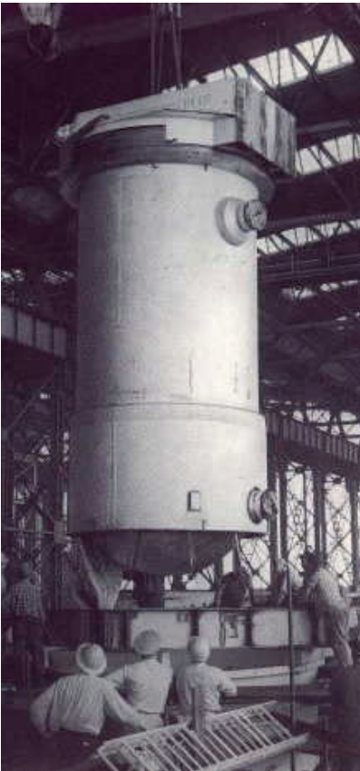
Figure 7-2 Reactor Vessel during Fabrication
