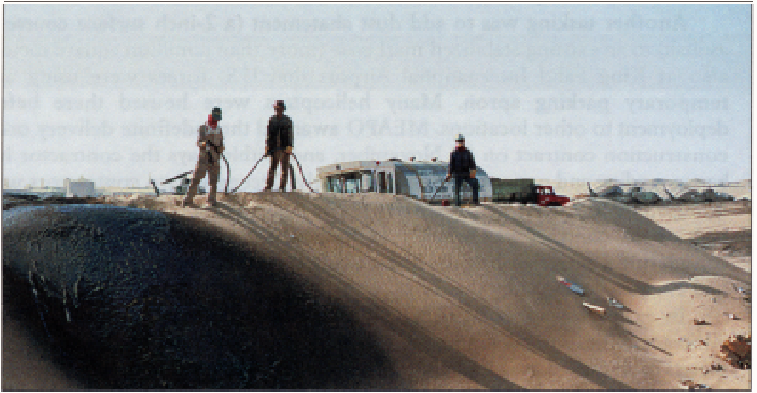
Hand application of dust palliative at Al Hasa.
