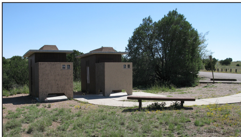
Aldo Leopold Vista restrooms
