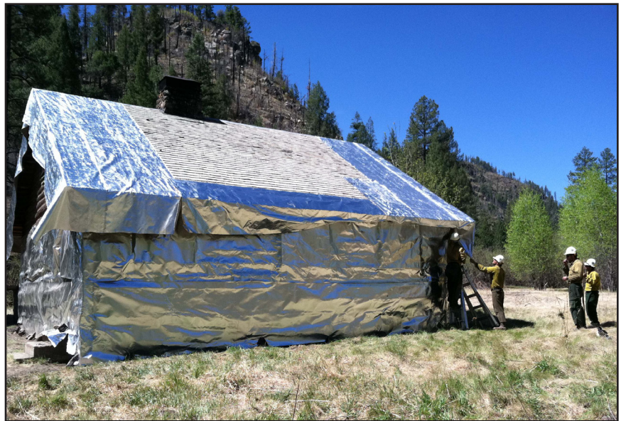
Protective wrapping at White Creek Cabin during the Miller Fire
