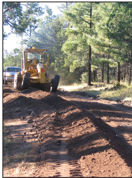
Rehab and maintenance work on FR 150
