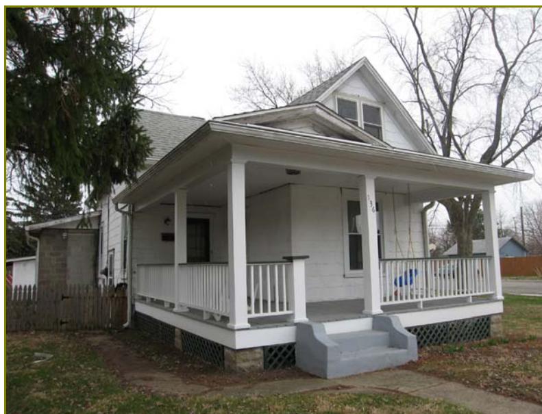
Figure 19. 136 W. Dayton Drive, looking southwest
