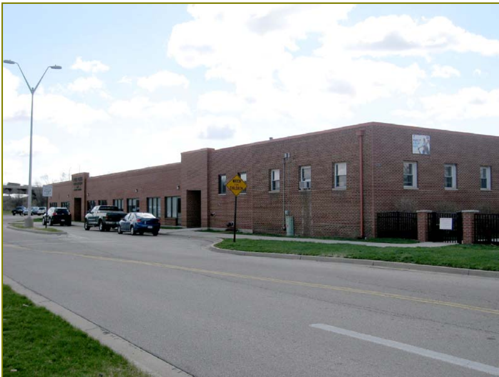
Photo 71. 300 S. Central Avenue, looking southeast
