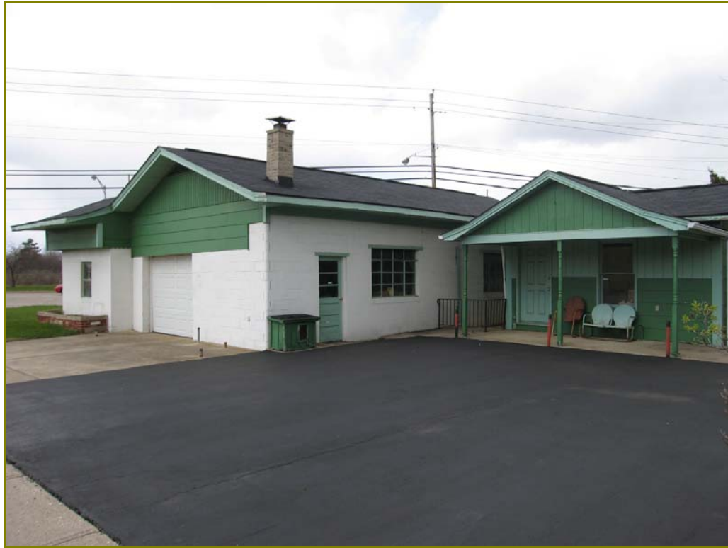
Photo 15. 435 Vine Street, looking northwest
