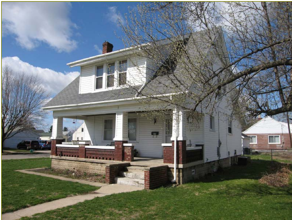
Photo 88. 121 S. Central Avenue, looking southwest
