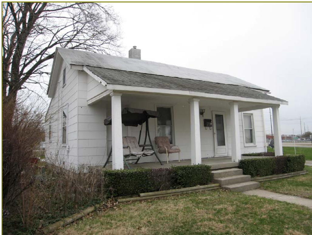
Photo 191. 548 South Street, looking southwest
