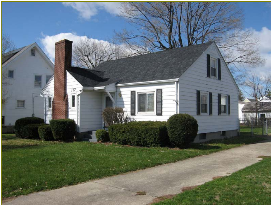
Photo 90. 117 S. Central Avenue, looking southwest
