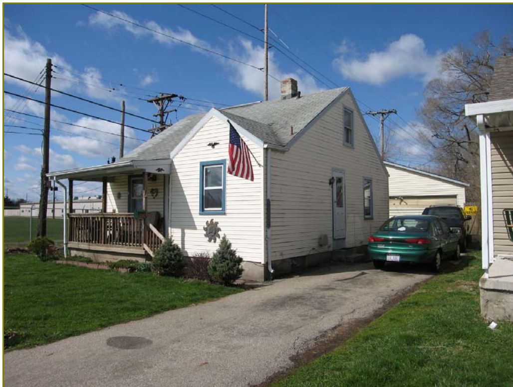
Photo 55. 409 S. Central Avenue, looking southwest
