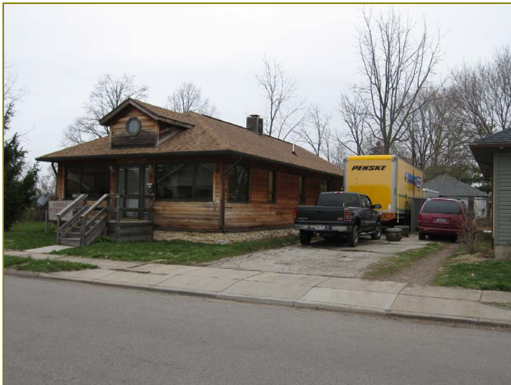
Photo 183. 529 Ohio Street, looking northwest
