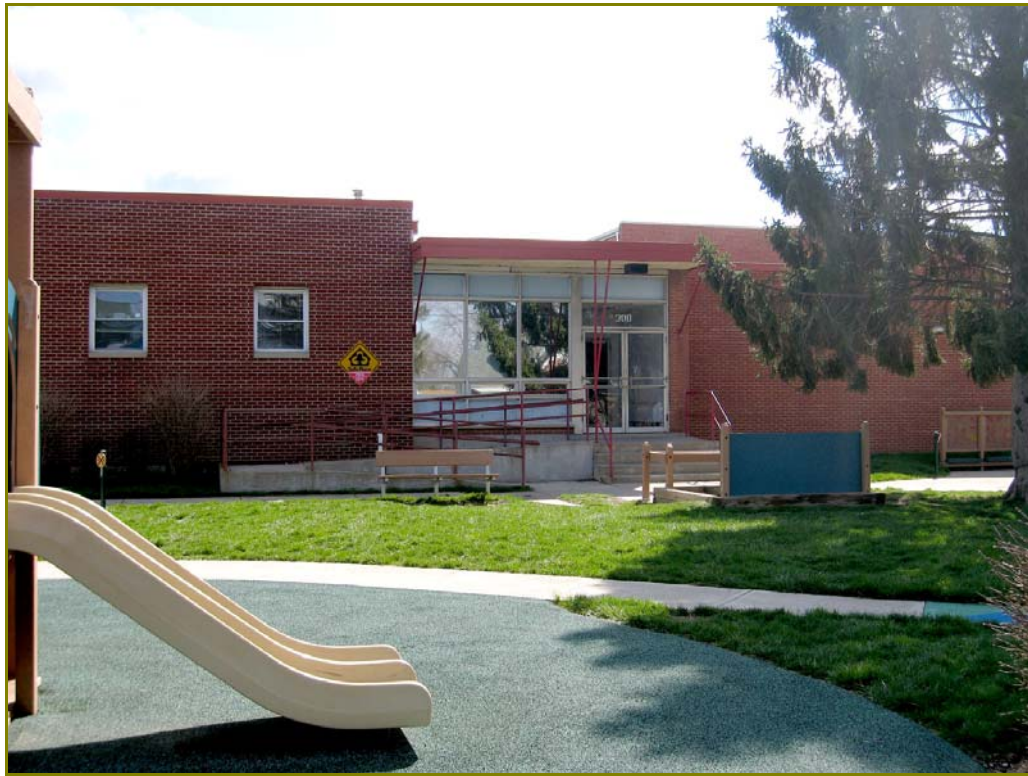
Photo 72. 300 S. Central Avenue, looking southeast
