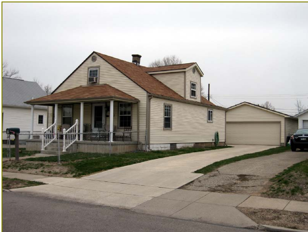
Photo 207. 531 South Street, looking northwest
