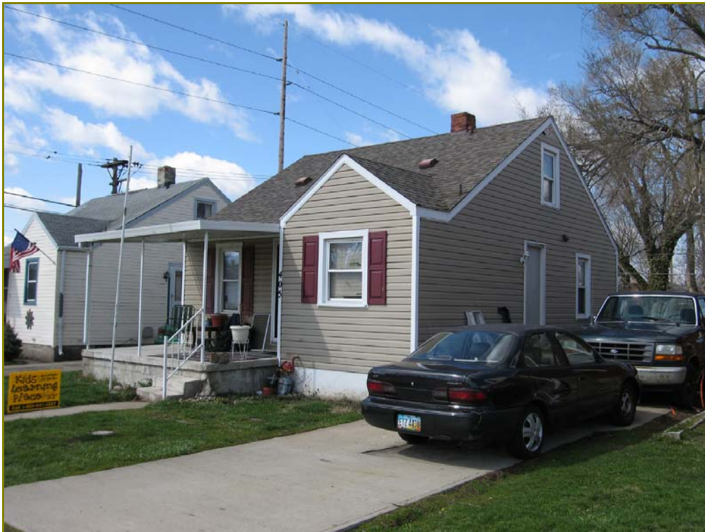
Photo 57. 405 S. Central Avenue, looking southwest
