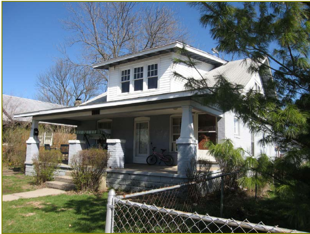
Photo 138. 311 W. Dayton Drive, looking northwest
