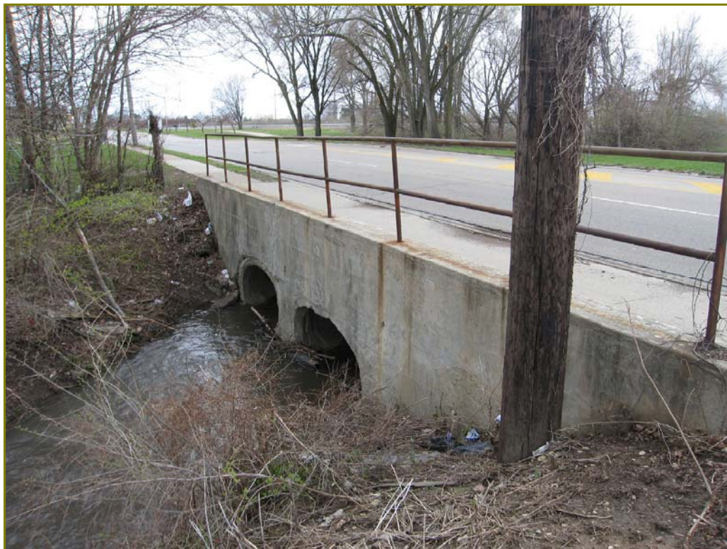
Photo 37. 900 block of Kauffman Avenue culvert, looking southwest
