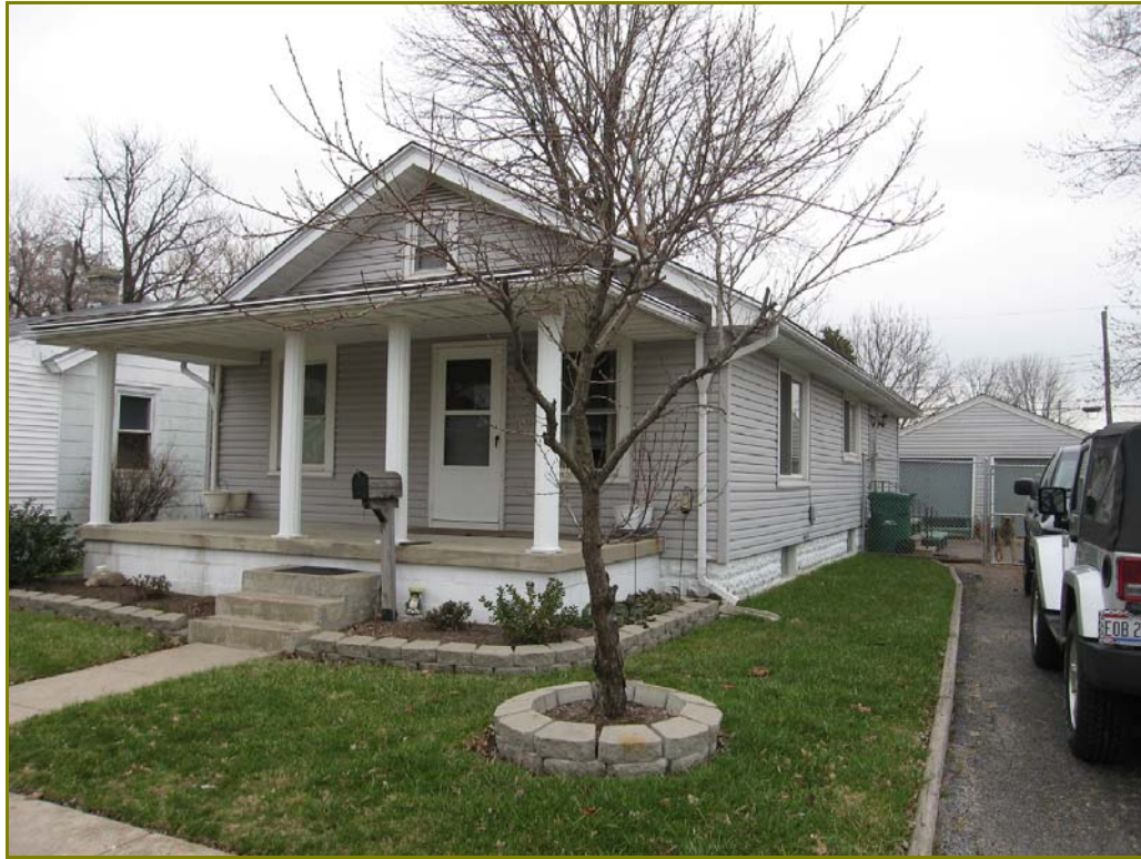
Photo 174. 514 Greene Street, looking southeast
