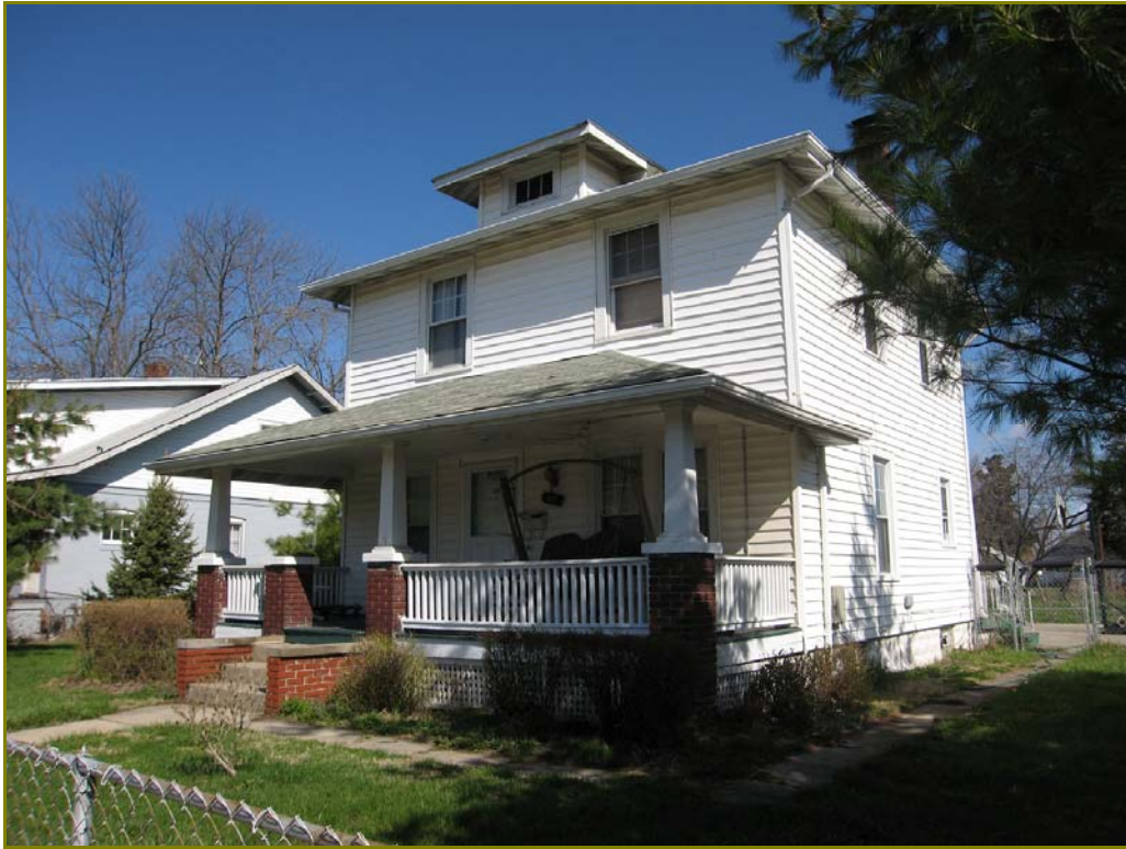
Photo 134. 307 W. Dayton Drive, looking northwest
