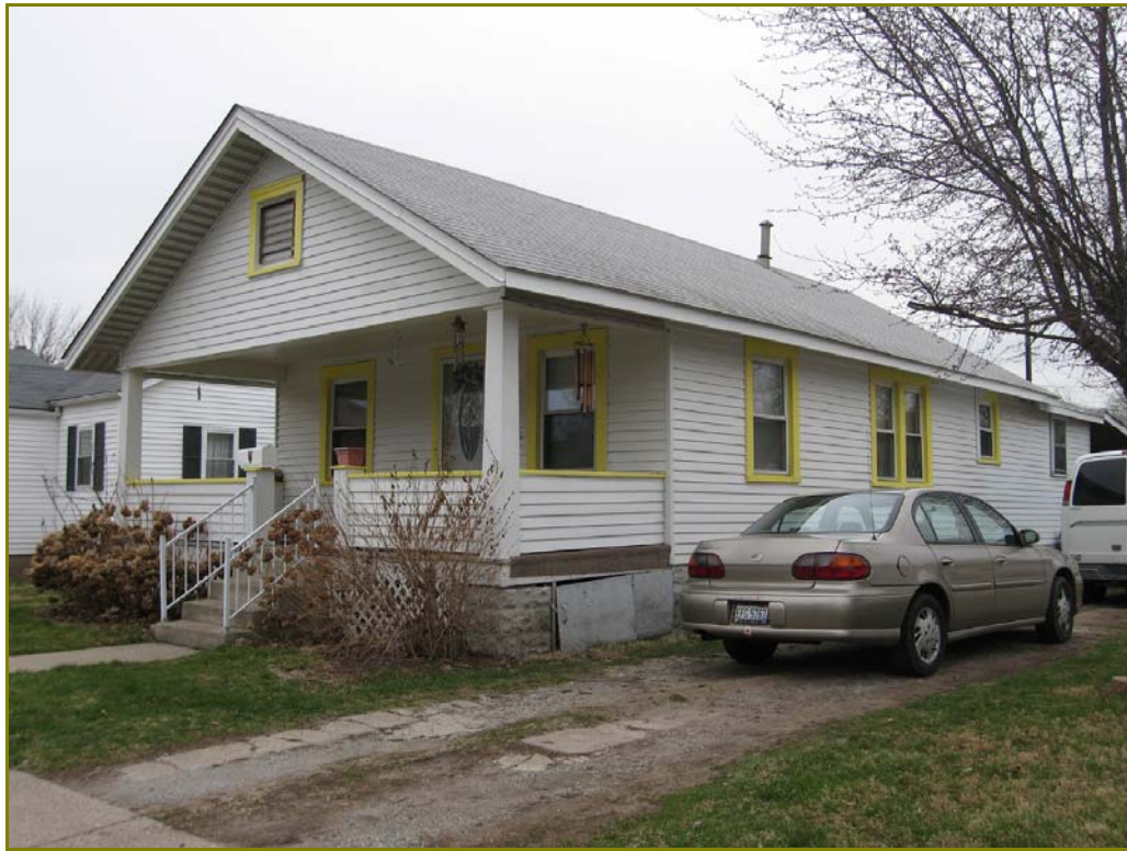
Photo 178. 534 Ohio Street, looking southeast
