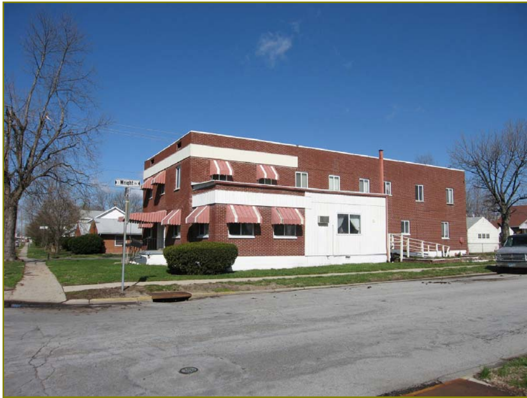
Photo 116. 201 W. Dayton Drive, looking northwest
