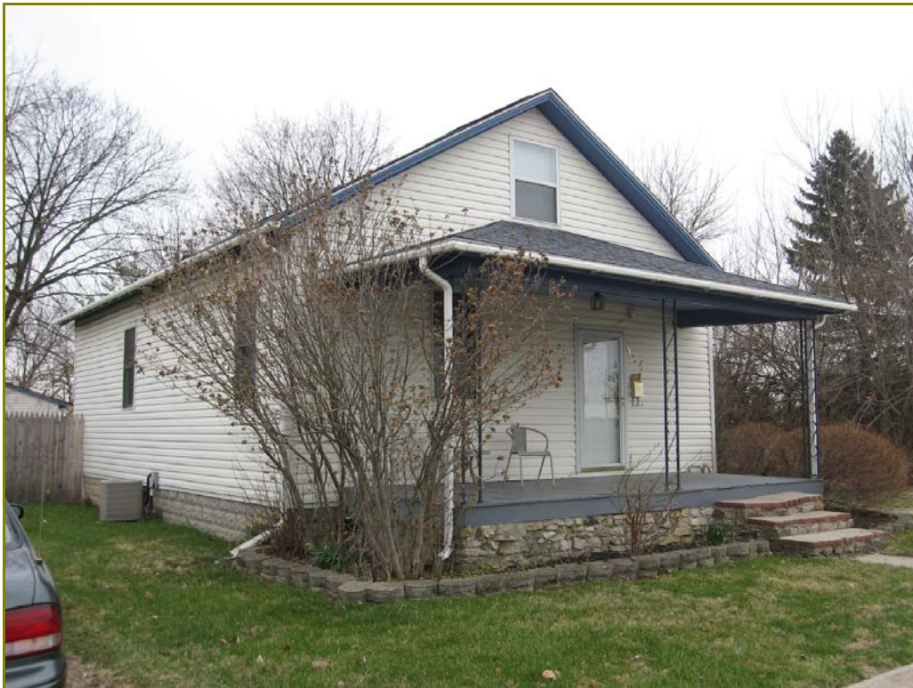
Photo 169. 528 Greene Street, looking southwest
