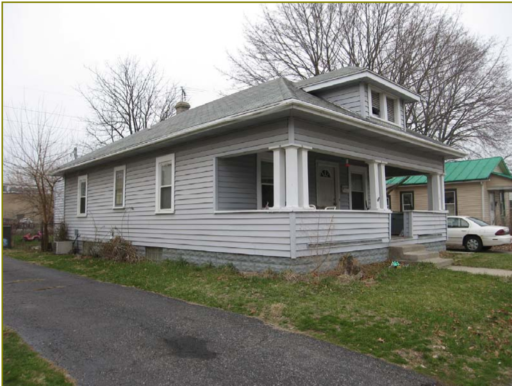
Photo 199. 540 South Street, looking southwest
