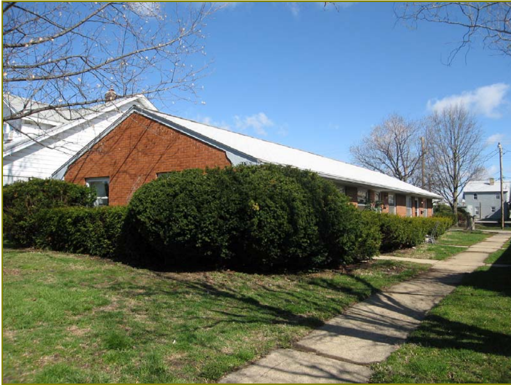
Photo 122. 213 W. Dayton Drive, looking northwest
