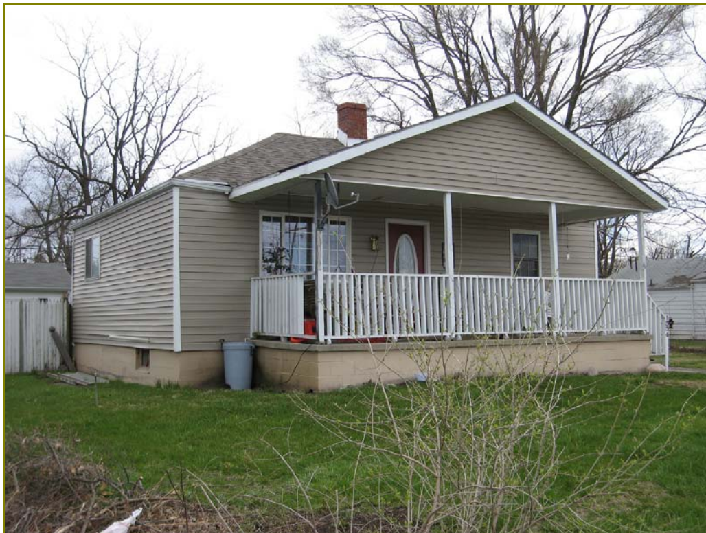
Photo 8. 1554 Montgomery Avenue, looking southeast
