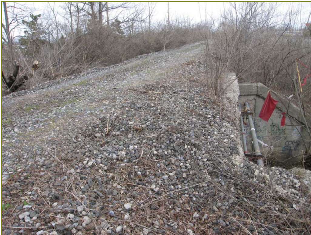
Photo 33. Railroad Bridge 2, looking northeast
