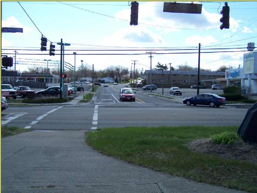
Photo 20. Area C: intersection of W. Garland Avenue and Kauffman Avenue, looking southeast
