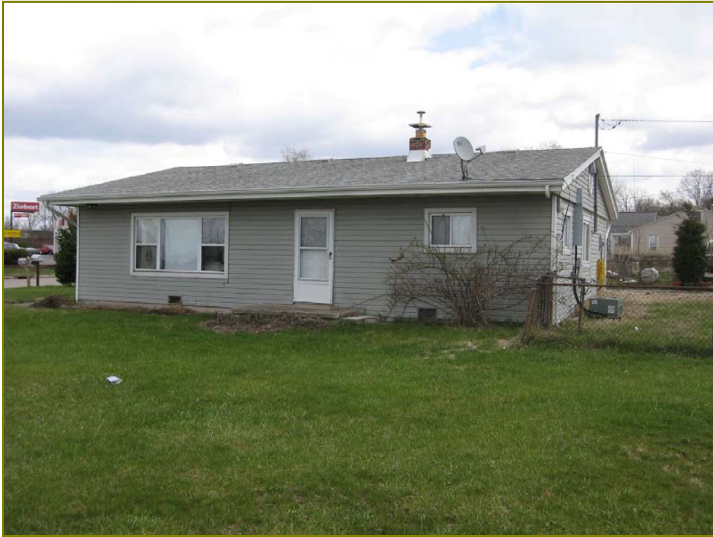
Photo 23. 408 West Gilbert Avenue, looking northeast
