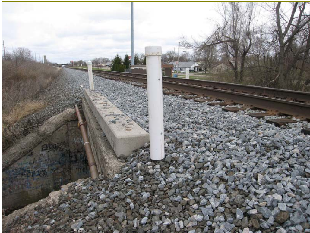
Photo 31. Railroad Bridge 1, looking northeast
