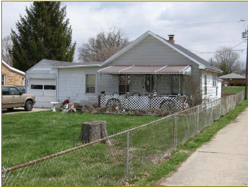
Photo 1. 1612 North Boulevard, looking northeast
