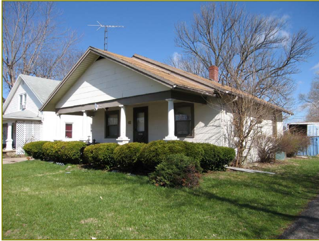
Photo 144. 403 W. Dayton Drive, looking northwest
