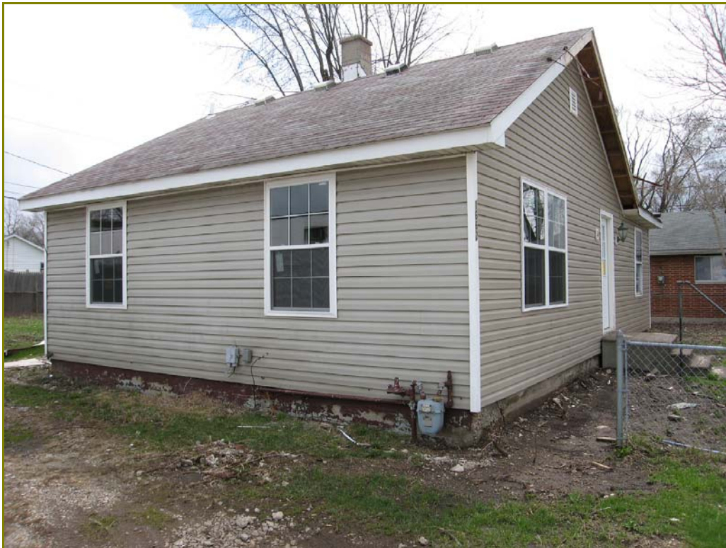
Photo 10. 1662 Kauffman Avenue, looking southeast
