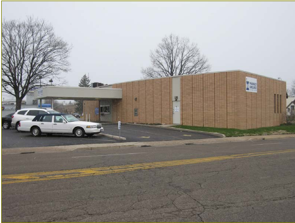
Photo 91. 77 S. Central Avenue (GRE-1212-10), looking northeast
