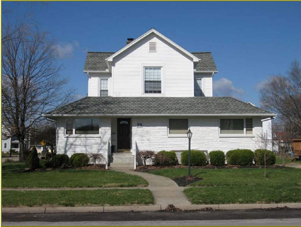
Photo 99. 75 S. Grand Avenue, looking west
