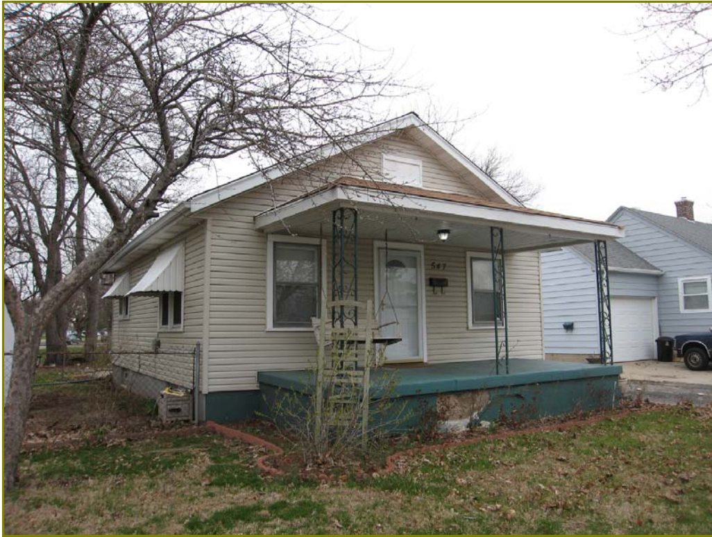
Photo 192. 547 South Street, looking northeast
