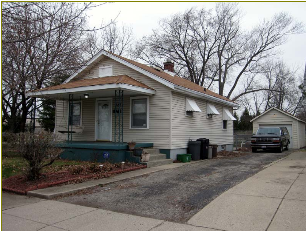
Photo 193. 547 South Street, looking northwest
