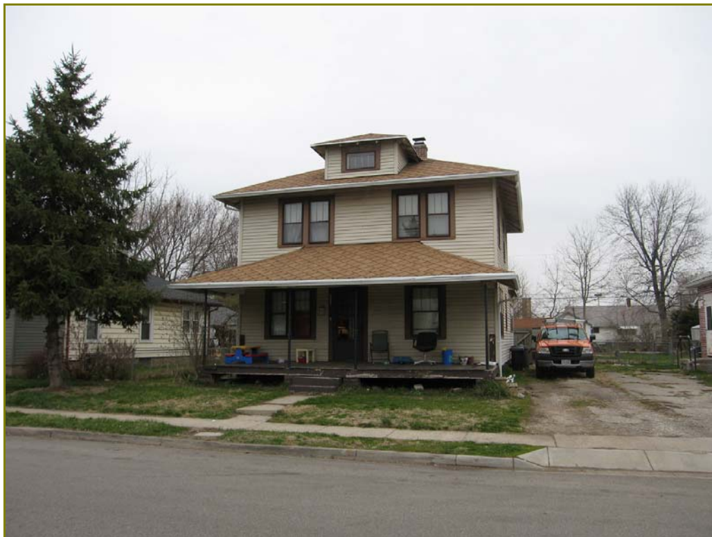
Photo 189. 521 Ohio Street, looking north
