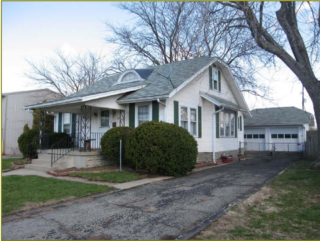
Photo 152. 411 W. Dayton Drive, looking northwest
