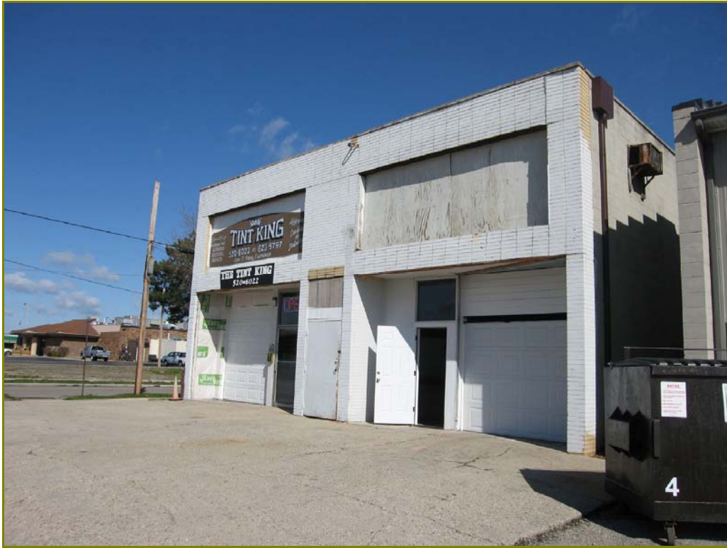
Photo 156. 417 W. Dayton Drive, looking northwest
