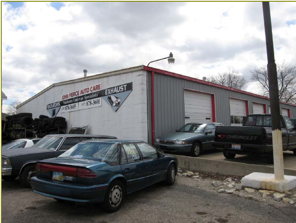
Photo 47. 808 Kauffman Avenue, looking southeast
