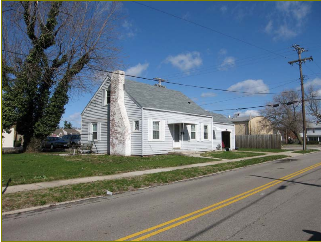
Photo 160. 53 Second Street, looking northwest
