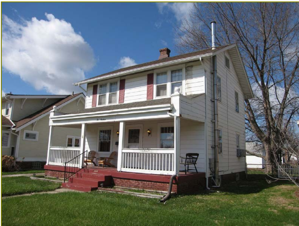
Photo 80. 219 S. Central Avenue, looking southwest
