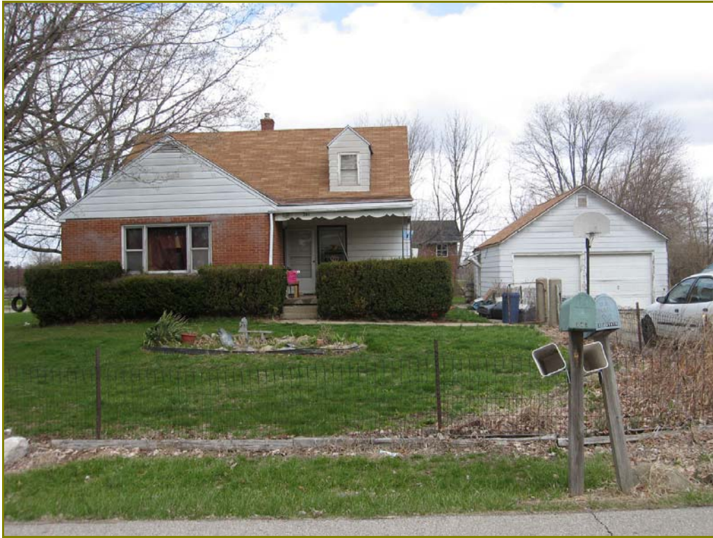
Photo 26. 341 State Street, looking north
