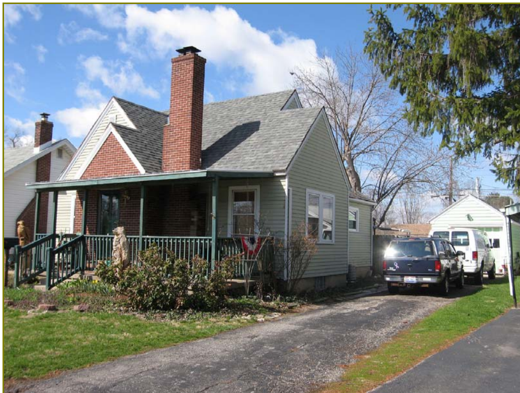
Photo 65. 313 S. Central Avenue, looking southwest
