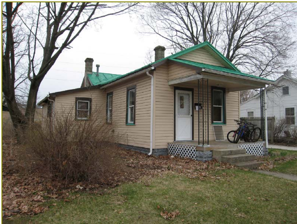
Photo 195. 544 South Street, looking southwest
