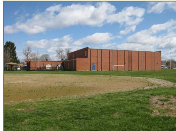
Figure 40. 300 S. Central Avenue, looking northeast at the Fairborn YMCA
