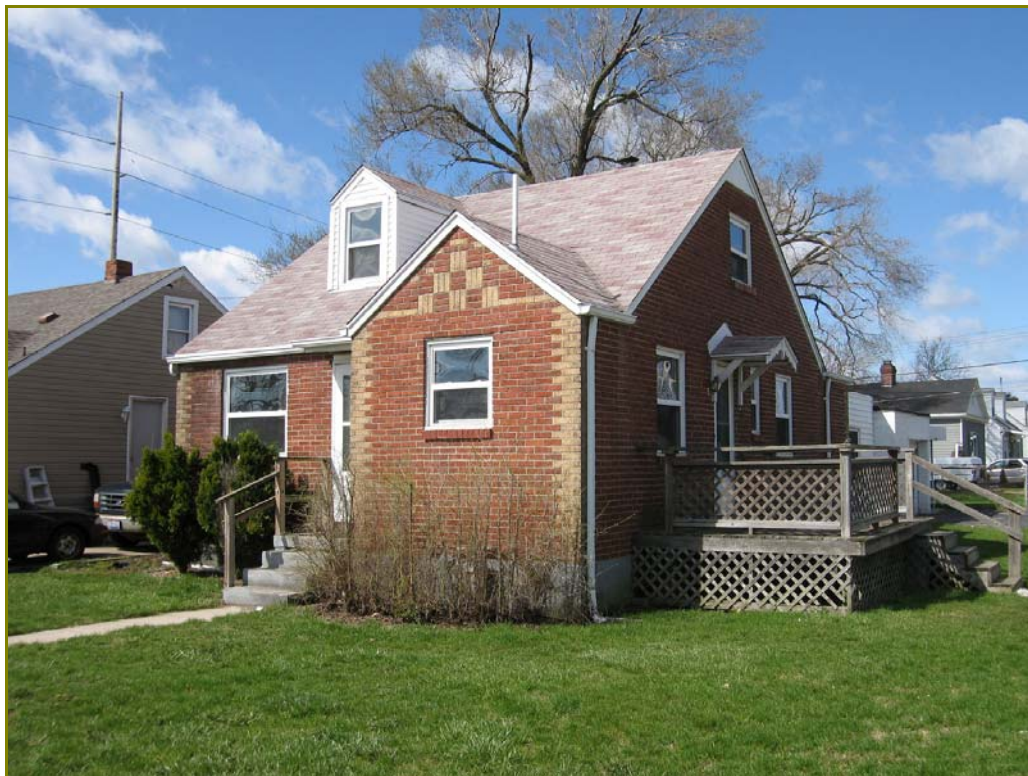
Photo 59. 401 S. Central Avenue, looking southwest
