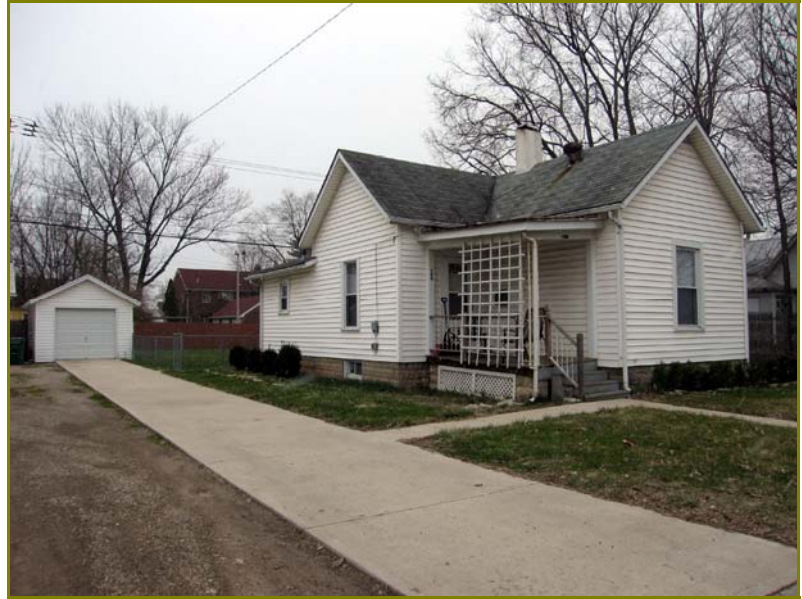
Figure 16. 104 W. Dayton Drive, looking southwest
