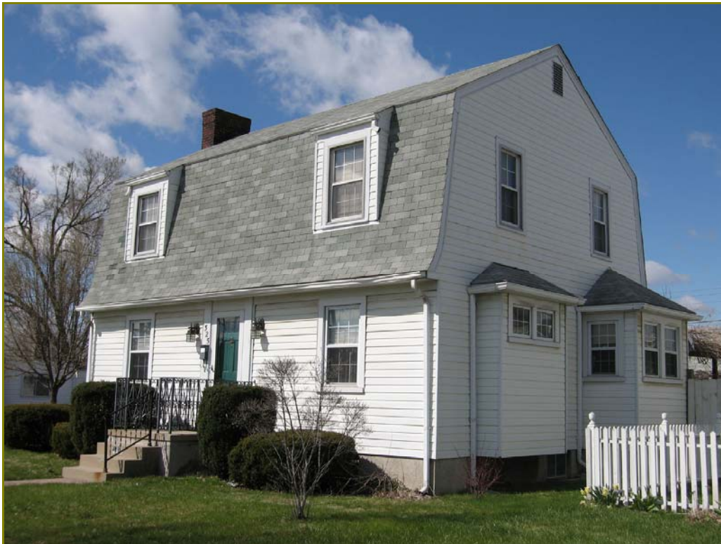
Photo 61. 325 S. Central Avenue, looking southwest
