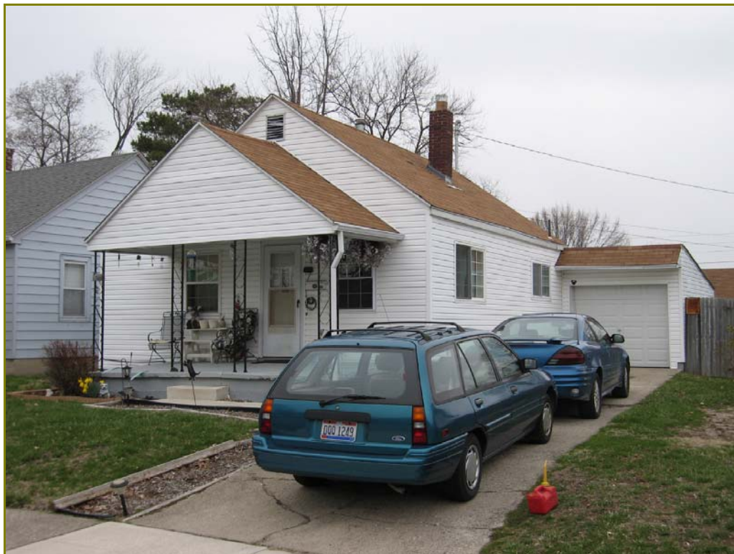
Photo 201. 539 South Street, looking northwest
