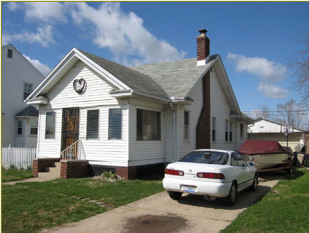
Photo 63. 319 S. Central Avenue, looking southwest
