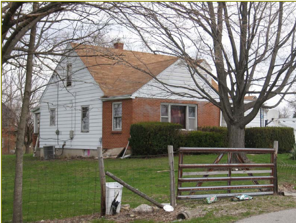
Photo 27. 341 State Street, looking northeast
