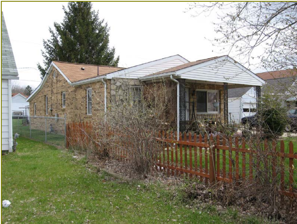
Photo 4. 1608 North Boulevard, looking southeast
