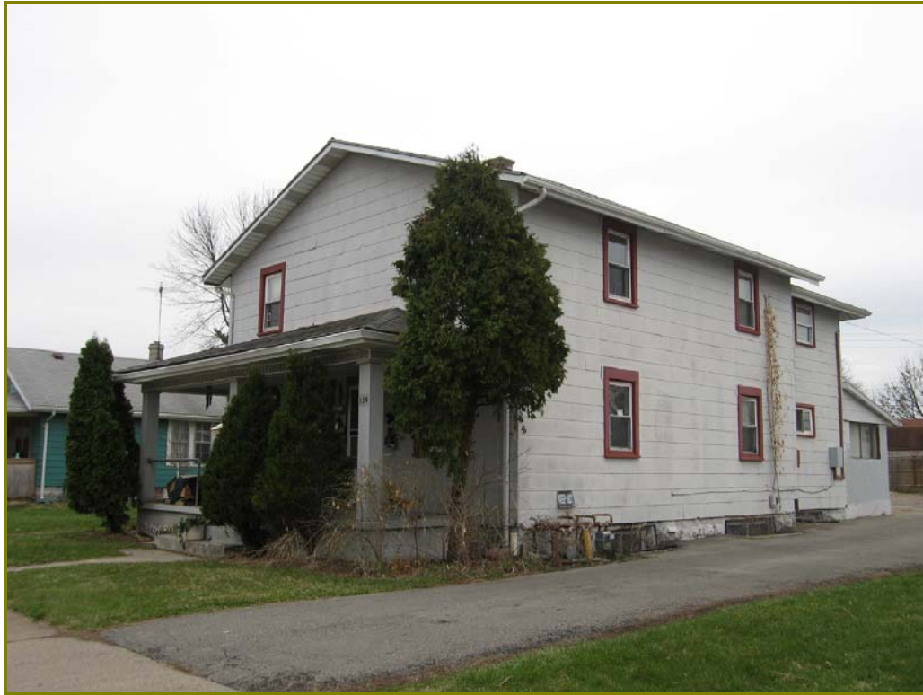
Photo 186. 522-524 Ohio Street, looking southeast
