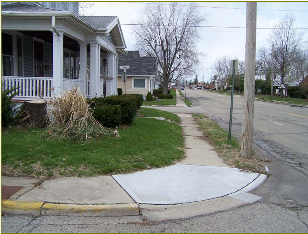
Photo 39. Area E: intersection of W. Dayton Drive and S. Wright Avenue, looking west
