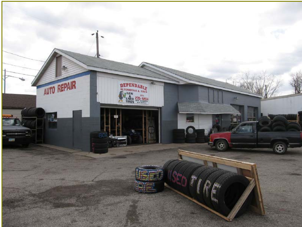
Photo 49. 806 Kauffman Avenue, looking southeast
