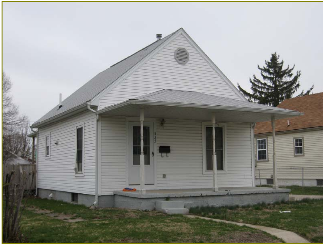
Photo 204. 535 South Street, looking northeast
