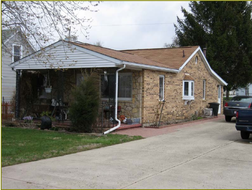
Photo 3. 1608 North Boulevard, looking northeast
