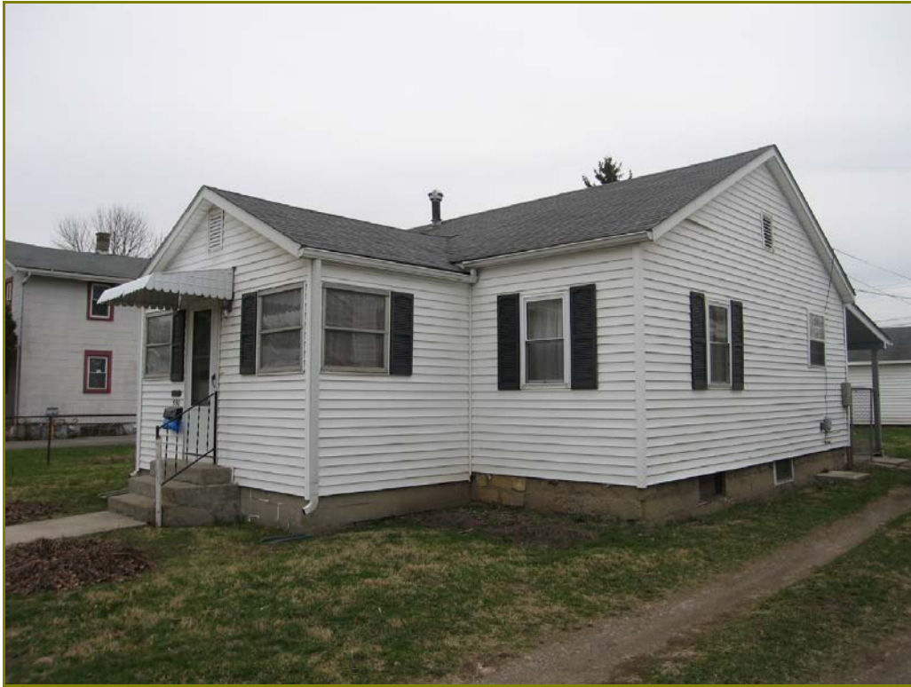
Photo 180. 530 Ohio Street, looking southeast
