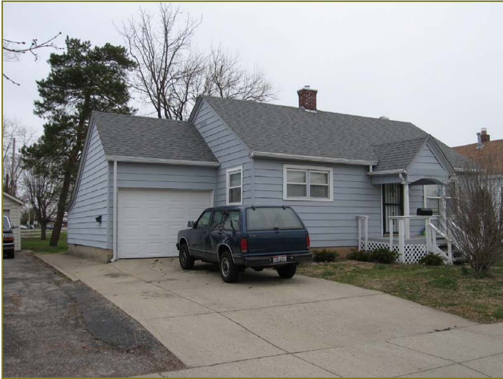
Photo 196. 543 South Street, looking northeast
