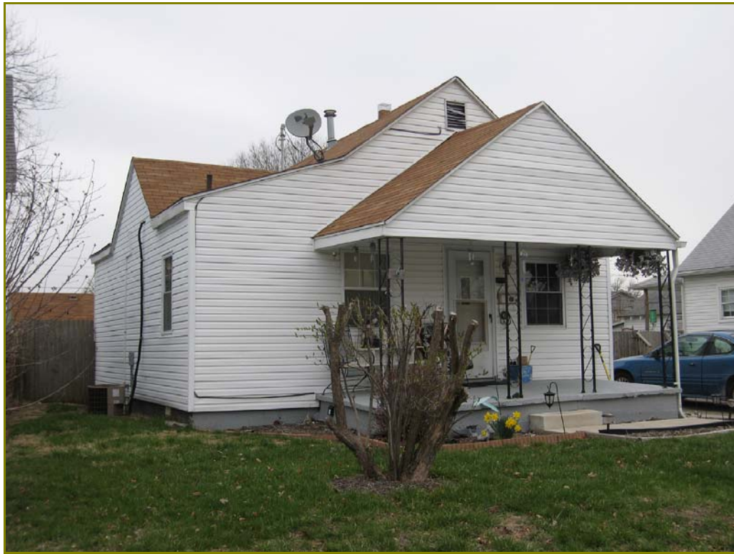
Photo 200. 539 South Street, looking northeast
