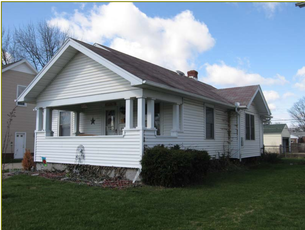
Photo 84. 207 S. Central Avenue, looking southwest
