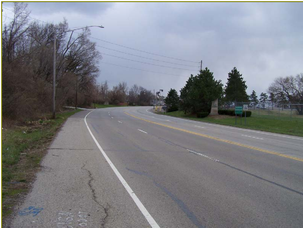
Photo 52. Area G: view along east side of SR 235, looking south
