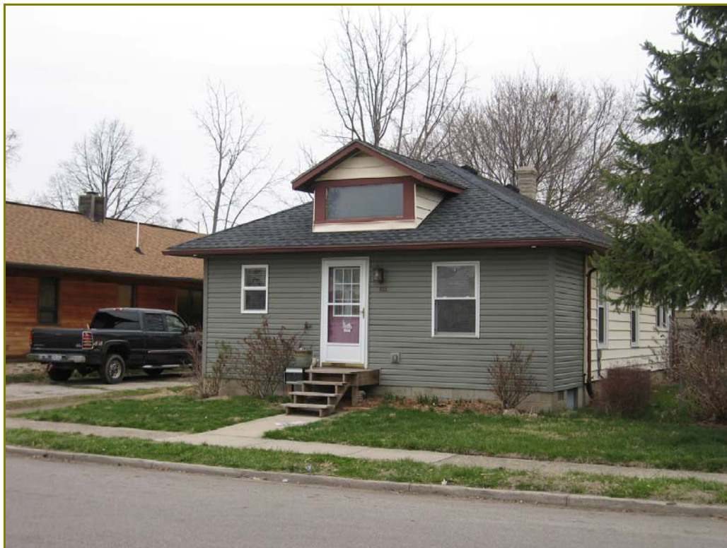
Photo 185. 525 Ohio Street, looking northwest
