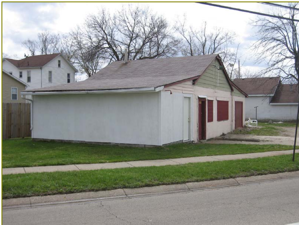
Photo 45. 824 Kauffman Avenue, looking southeast
