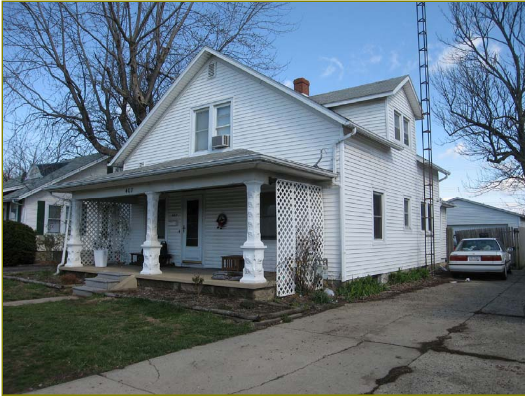
Photo 148. 407 W. Dayton Drive, looking northwest
