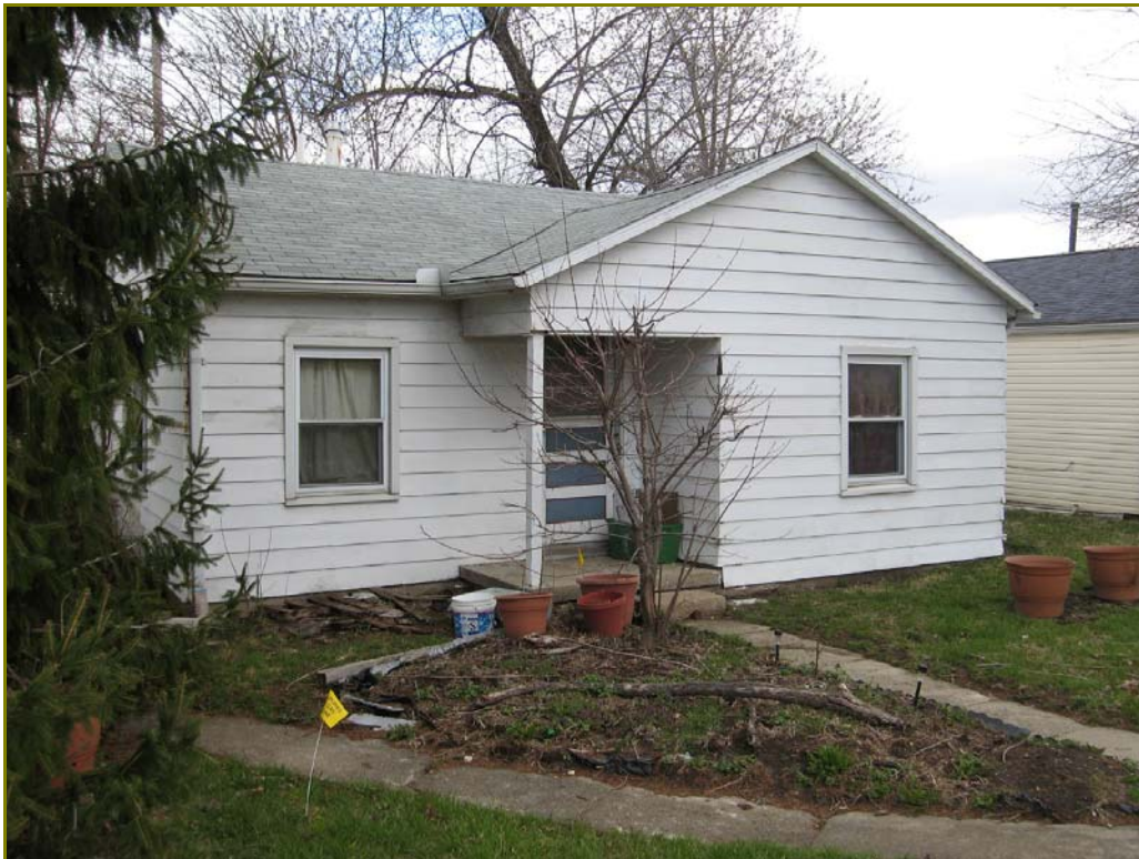
Photo 20. 423 Madison Street, looking northeast
