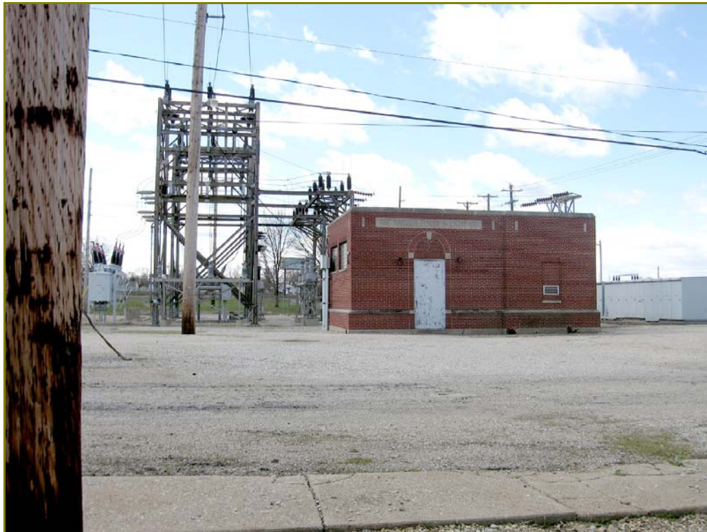
Photo 53. 410 S. Central Avenue, looking southwest
