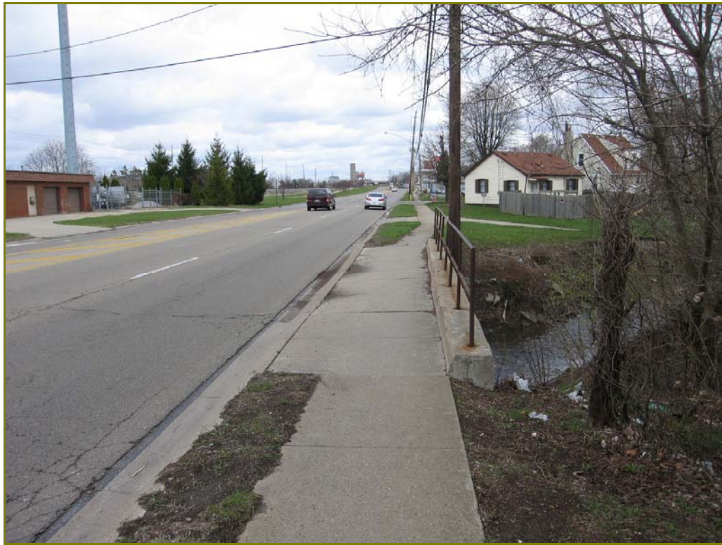
Photo 36. 900 block of Kauffman Avenue culvert, looking northeast
