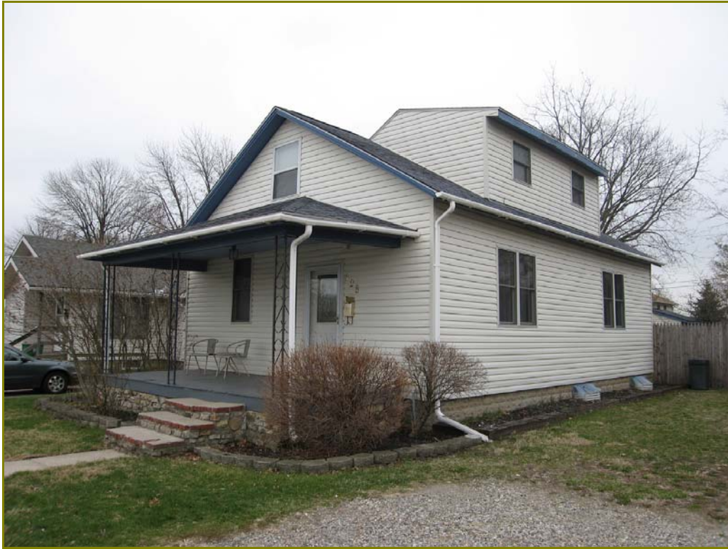
Photo 168. 528 Greene Street, looking southeast
