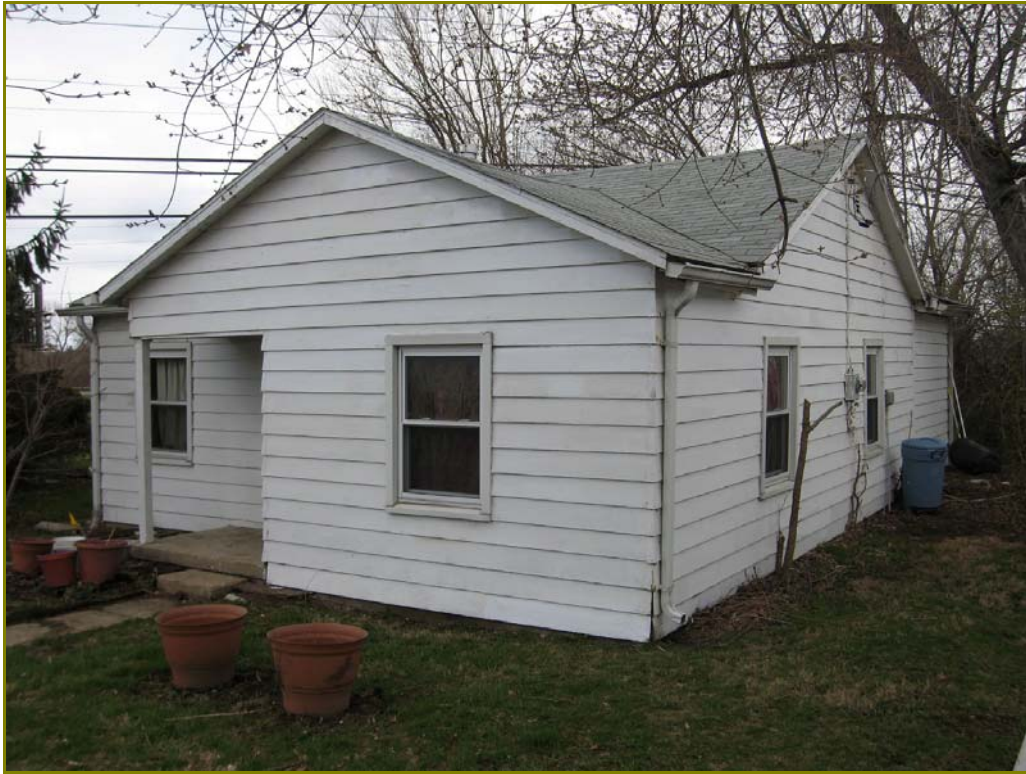
Photo 19. 423 Madison Street, looking northwest
