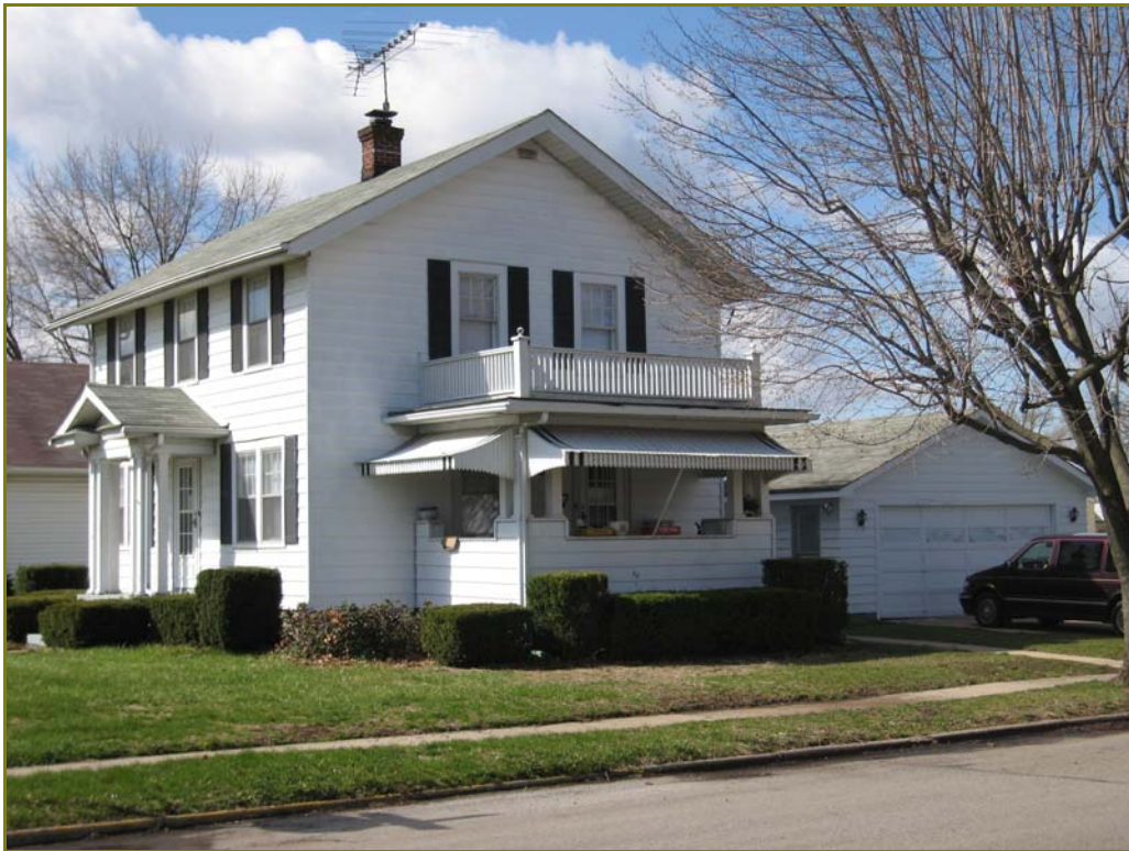
Photo 86. 201 S. Central Avenue, looking southwest
