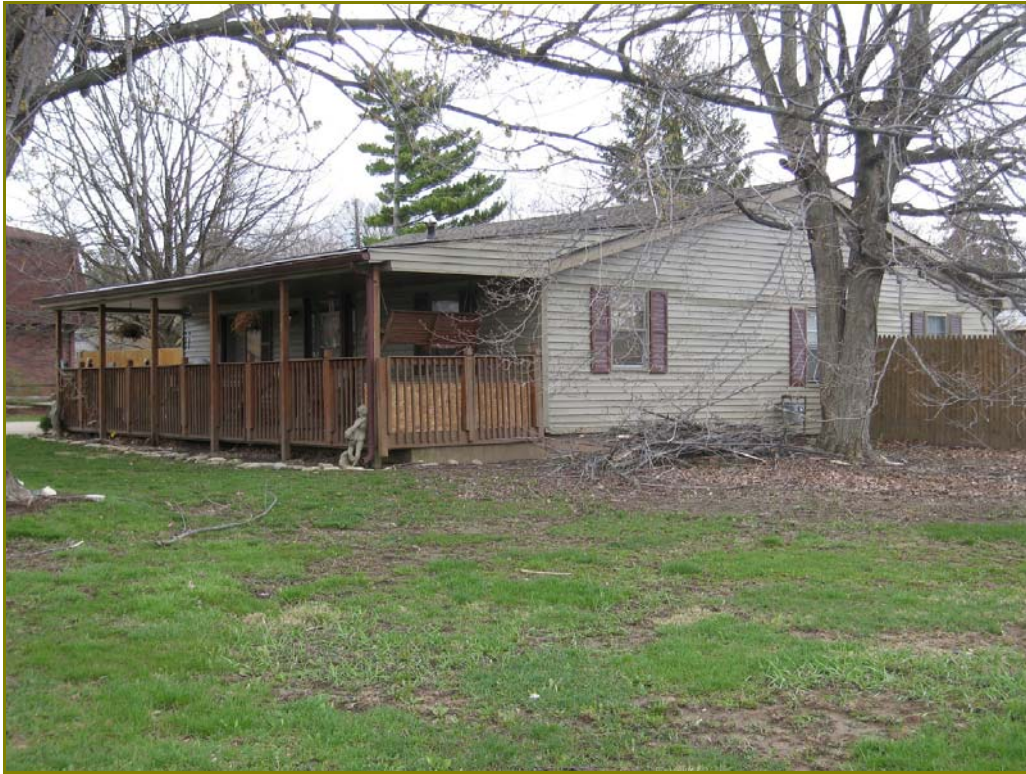
Photo 17. 424 Madison Street, looking southeast
