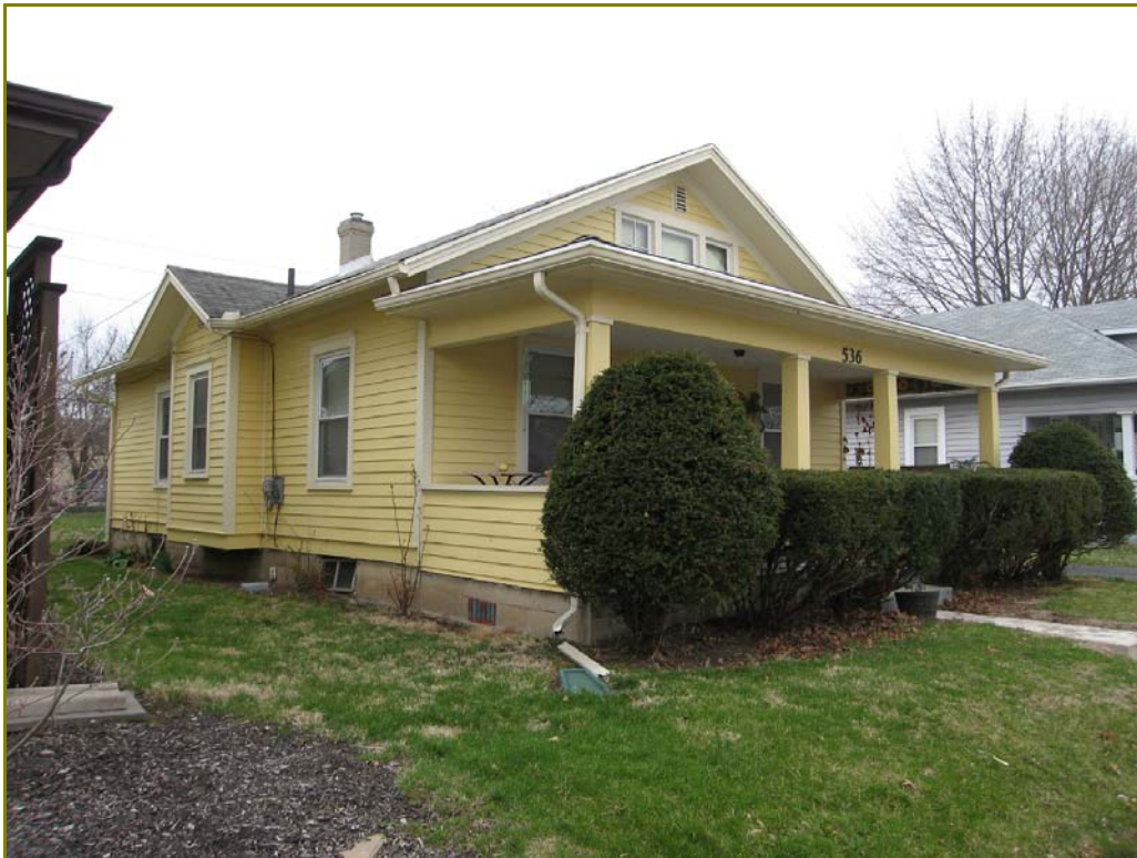
Photo 203. 536 South Street, looking southwest
