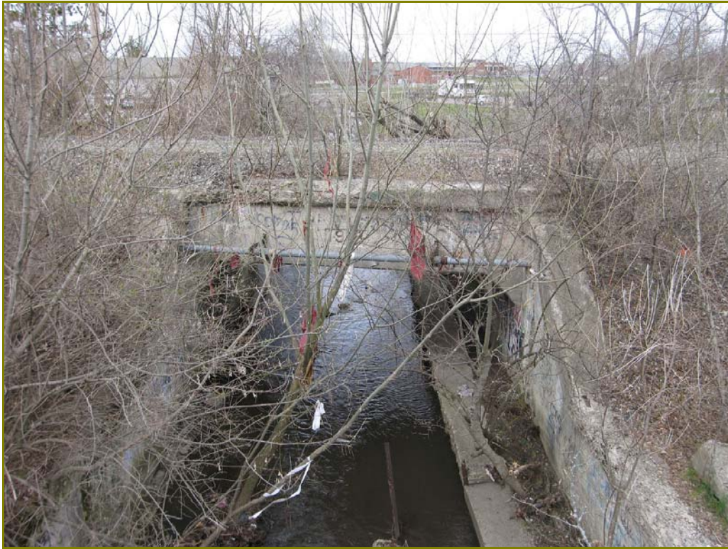
Photo 32. Railroad Bridge 2, looking northwest
