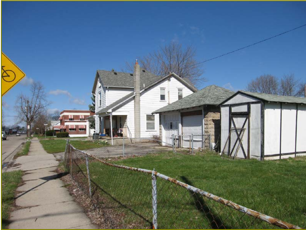
Photo 108. 127 W. Dayton Drive, looking northwest (GRE-246-10)
