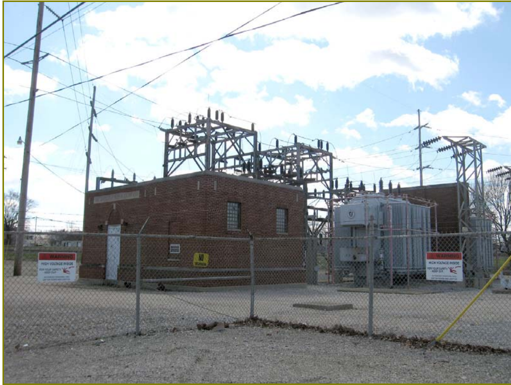
Photo 52. 410 S. Central Avenue, looking south
