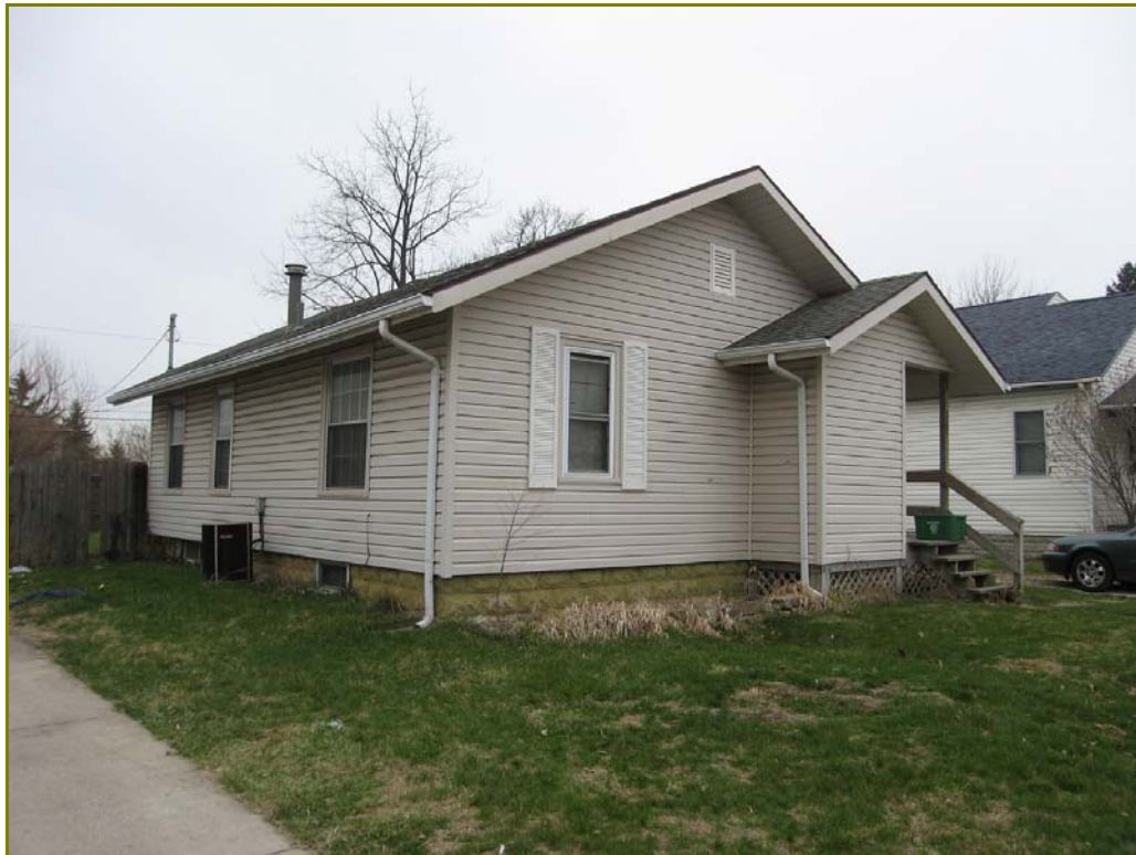
Photo 171. 520 Greene Street, looking southwest
