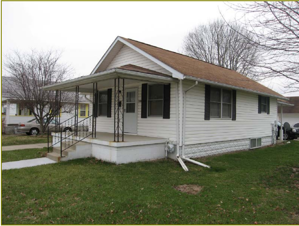
Photo 176. 538 Ohio Street, looking southeast
