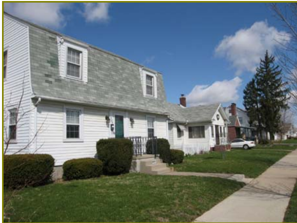
Figure 39. View of S. Central Avenue, looking northwest
