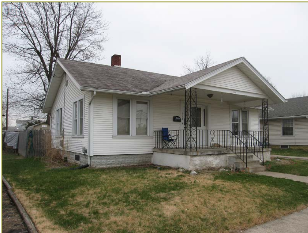
Photo 173. 518 Greene Street, looking southwest
