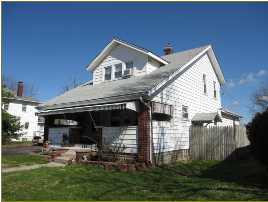
Photo 128. 219 W. Dayton Drive, looking northwest
