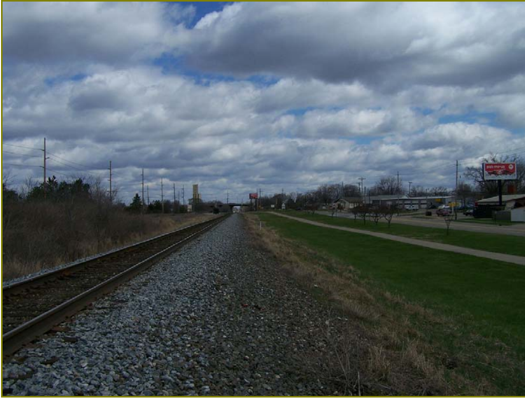
Photo 25. Area D: intersection of Kauffman Avenue and W. Lindberg Avenue, looking northeast
