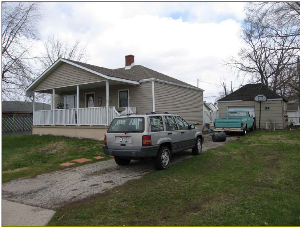
Photo 7. 1554 Montgomery Avenue, looking northeast
