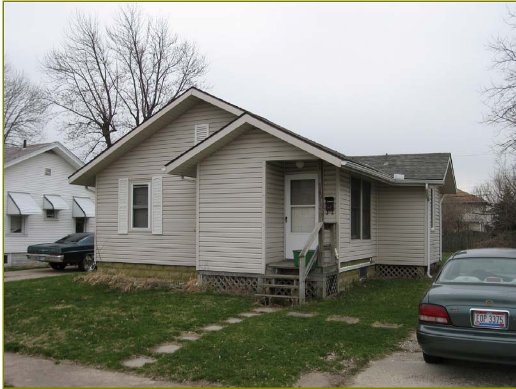
Photo 170. 520 Greene Street, looking southeast
