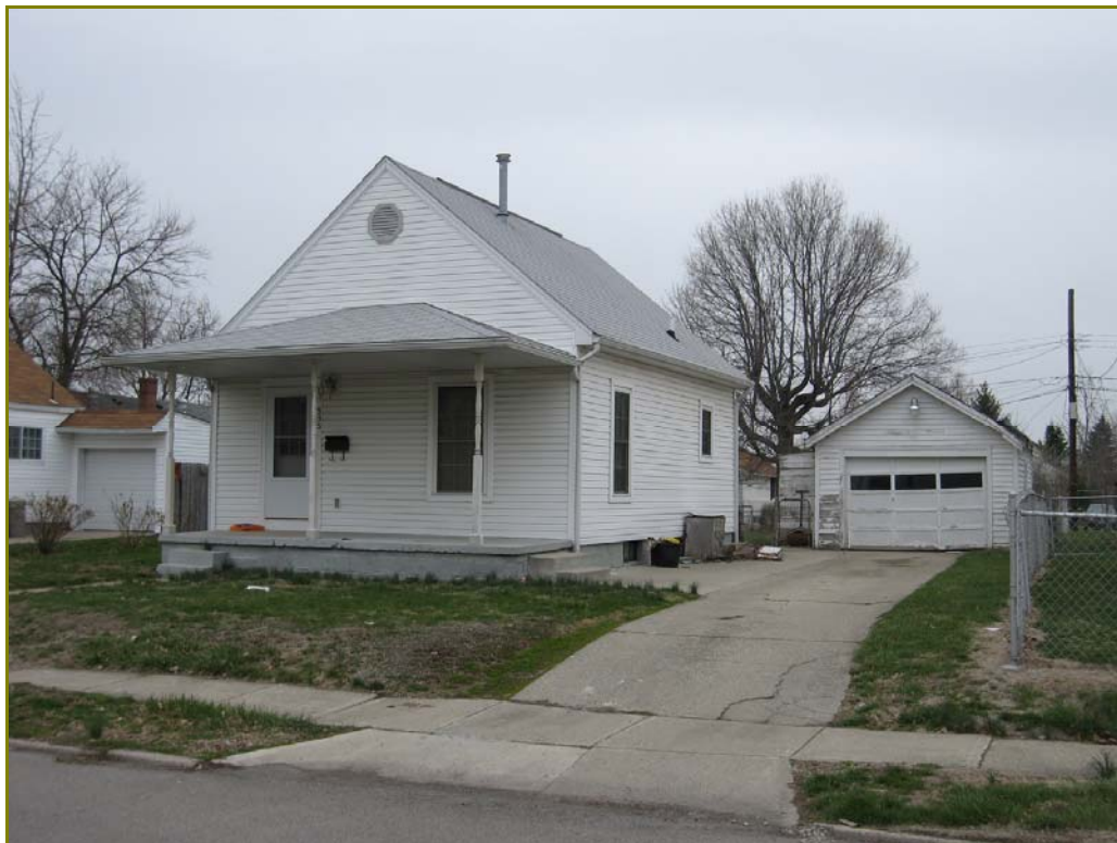
Photo 205. 535 South Street, looking northwest
