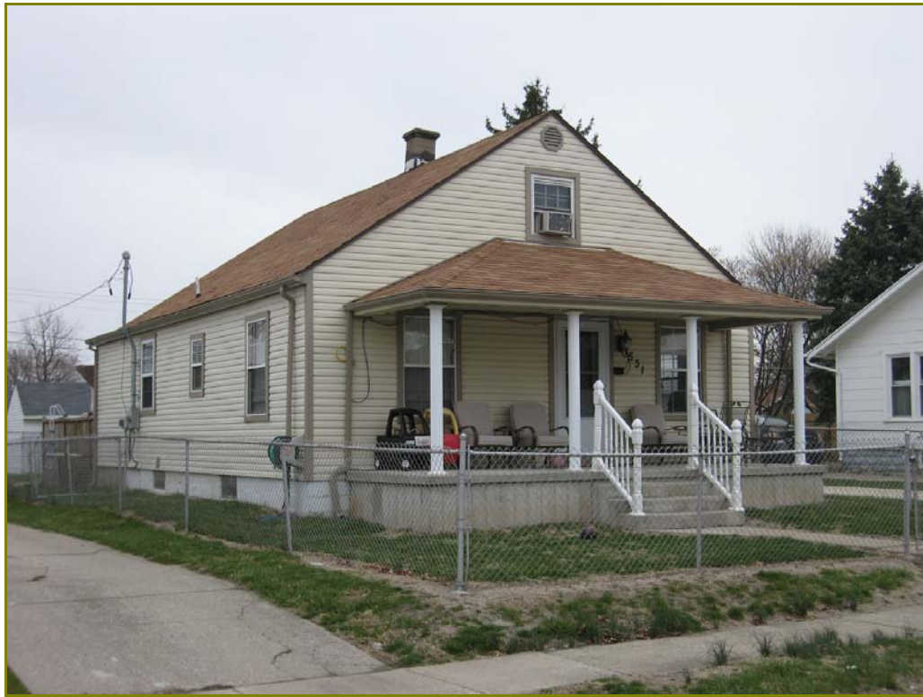
Photo 206. 531 South Street, looking northeast
