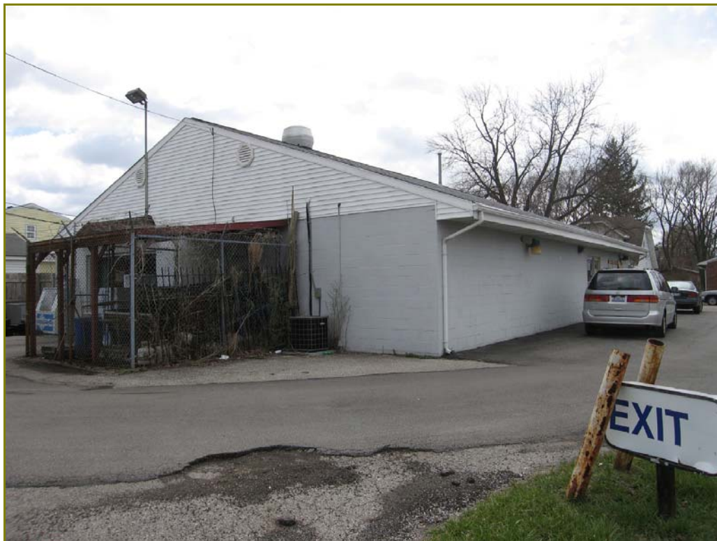
Photo 41. 868 Kauffman Avenue, looking southeast
