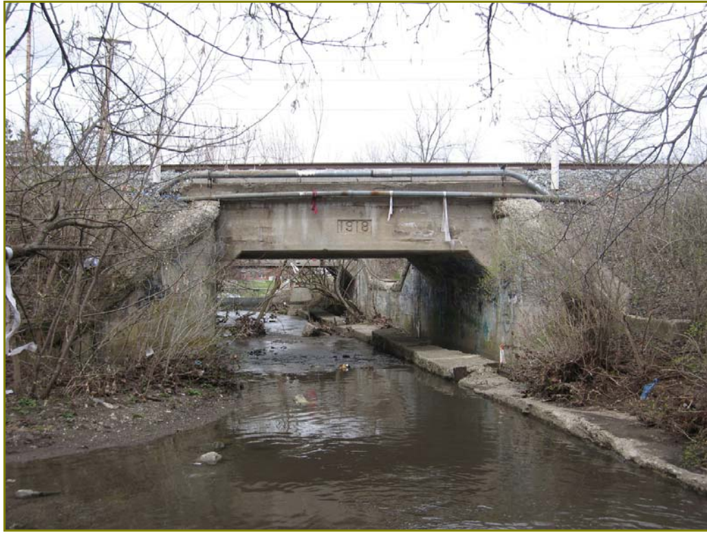
Photo 30. Railroad Bridge 1, looking northwest
