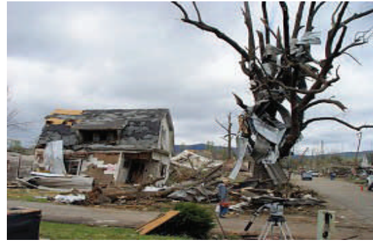
A tornado (rated EF3) ripped through this residential area, and wrapped metal around an oak tree Mena (Polk County) on 04/09/2009.
