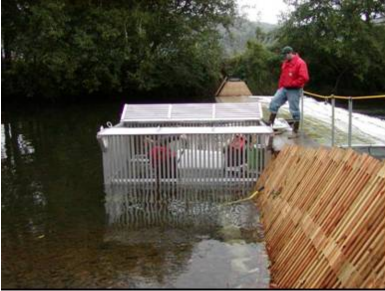
Figure 10 -- The Gray's River, WA weir, a resistance board/fixed panel design utilizing fixed wooden panels. Credit R. Walton.
