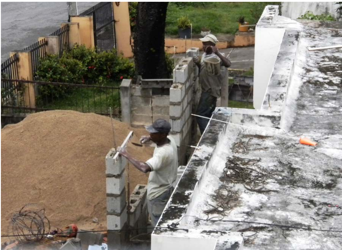
Image 1: Haitian block layers working on a residential project in Santo Domingo.
