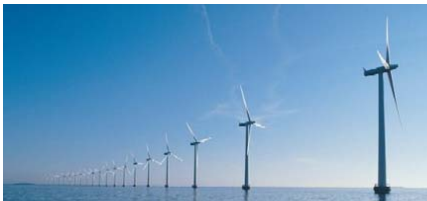
FIGURE 1 World’s First Offshore Wind Facility, Vindeby, Denmark, 1991 (Source: Siemens 2006)
