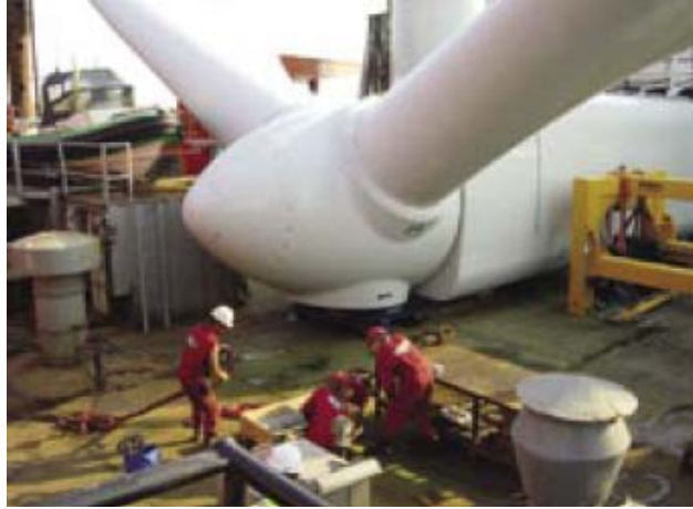
FIGURE 2 Rotor Assembly for Scroby Sands, United Kingdom Offshore Wind Facility (2-MW turbine) (Source: BWEA 2006c)
