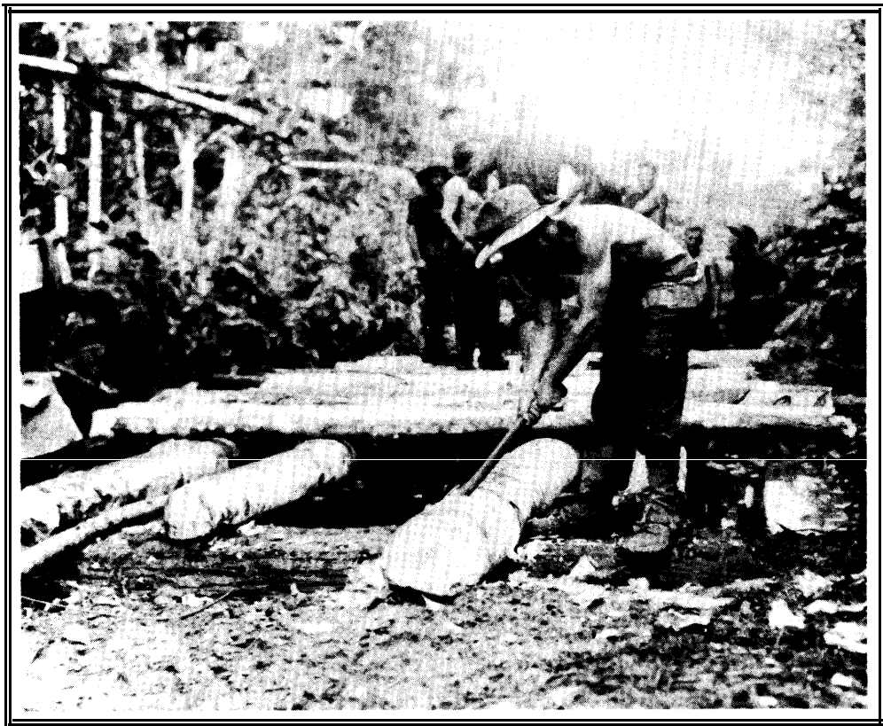
Corporal George Foster, 2d Pioneer Battalion, 7th Division, chops logs to fit into a bridge construction over a swampy area of road to Lao, New Guinea, 9 September 1943.
