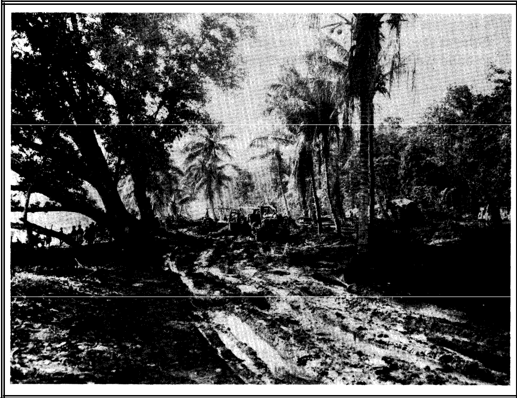
Muddy and rough roads made transportation difficult. Saidor, New Guinea, 18 January 1944.
