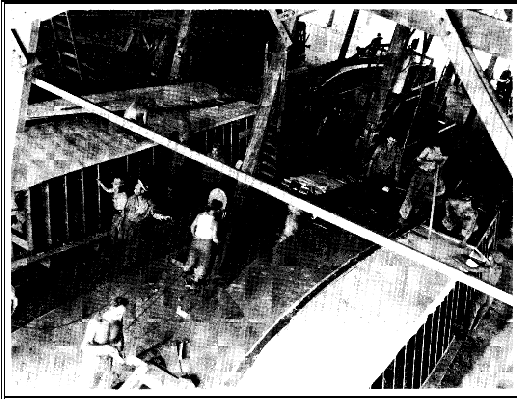
Assault boat construction by the 411th Engineer Battalion at Cairns, Queensland, Australia. Though the assembly plant is incomplete, building the Higgins boats has already started. 19 March 1943.
