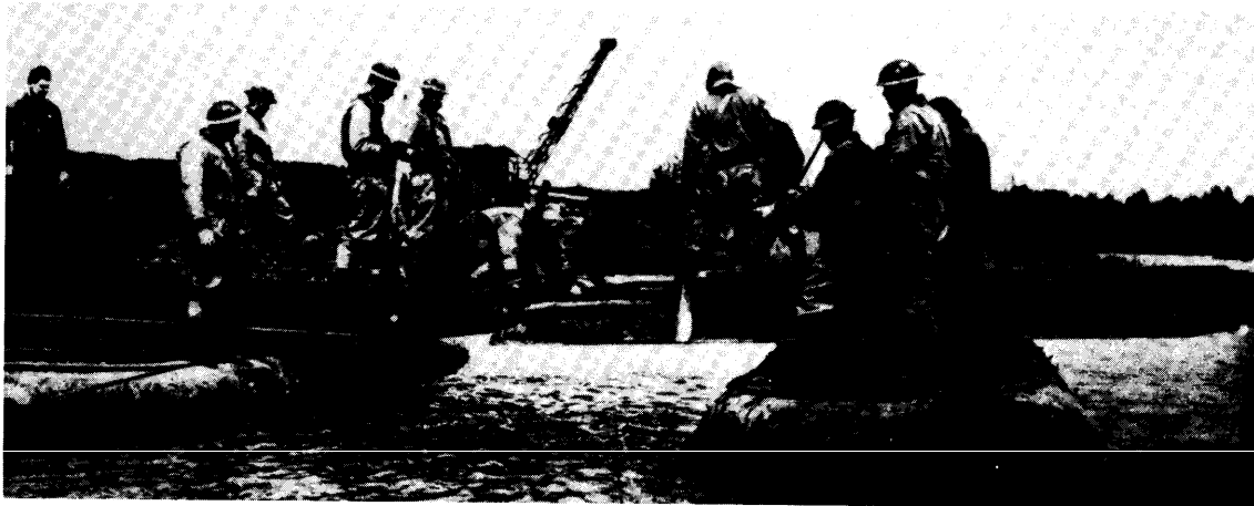
Tanks are Massive, Requiring Heavy Bridges for Their Movement
