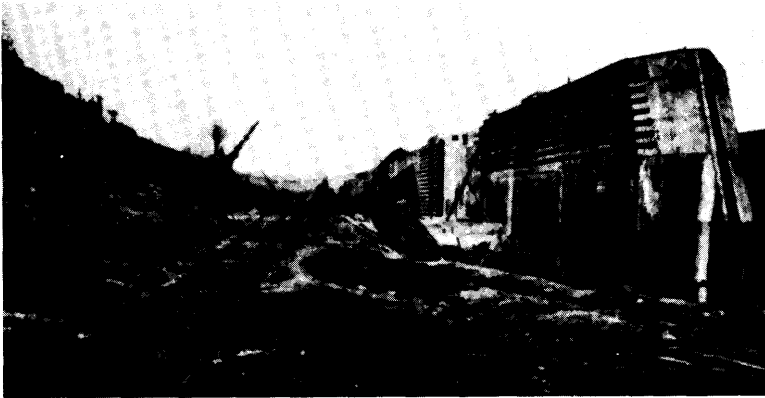
The Large Lock under Construction
