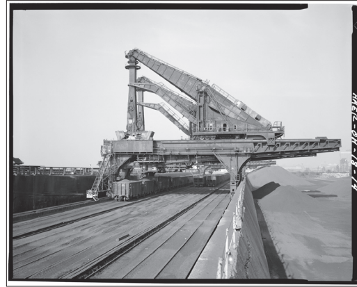
Massive Hulett Ore Unloaders are contributing elements to the historic Pennsylvania Railway Ore Dock. (Photo courtesy Library of Congress)
