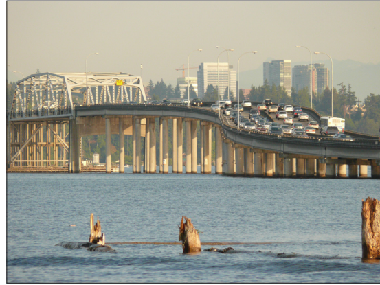
A portion of Evergreen Point Bridge viewed from the perspective of Lake Washington (Photo courtesy Washington Department of Transportation)
