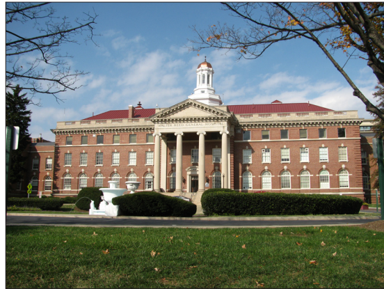
Walter Reed Army Medical Center's Building 1 will be part of the District of Columbia's land use redevelopment plan. (Photo courtesy U.S. Army Corps of Engineers, Fort Worth District)
