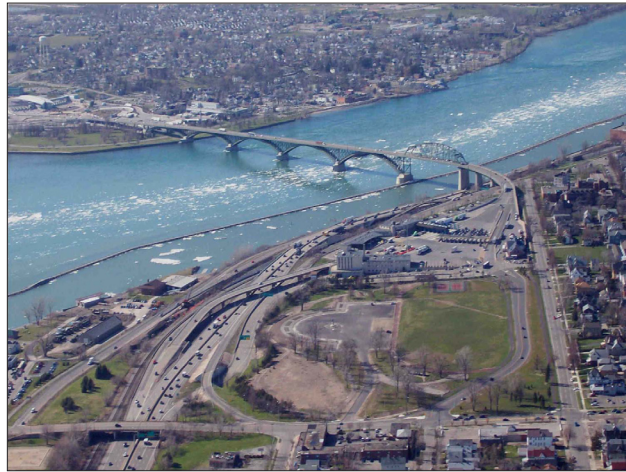
The Peace Bridge across the Niagara River dates to 1927. Canada is across the river at the top of this image. (Photo courtesy Federal Highway Administration)
