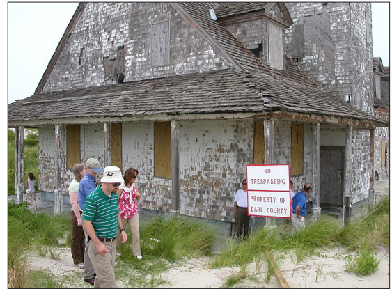
Former Coast Guard Station at Oregon Inlet prior to restoration
