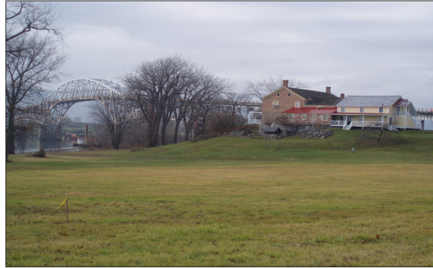
The former Lake Champlain Bridge from Chimney Point, Vermont, area. Note yellow archaeology pin flag in foreground near left bottom corner. (Photo courtesy Vermont Division for Historic Preservation)
