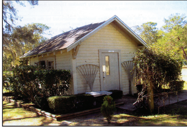
Building 1553, Camp Pinchot, Fort Walton Beach, Florida (photo: U.S. Air Force)
