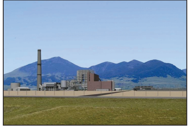
Artists rendition of the proposed Highwood Generation Station near the Great Falls Portage National Historic Landmark District, Great Falls, Montana. Image Courtesy of USDA Rural Utilities Service.
