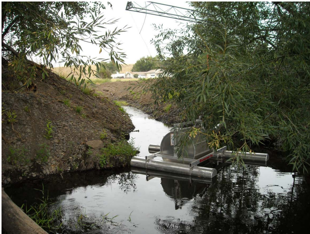
Figure 26. Photograph of the water diversion pump near the mouth of Doan Creek at WHMI.
