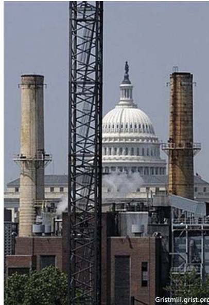
A coal-fired power plant (foreground) in Washington, D.C., emits particulate (soot) pollution to surrounding neighborhoods.
