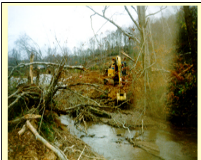
Fig. D.2-2 Backhoe Removing Woody Debris, Hall County, Georgia
