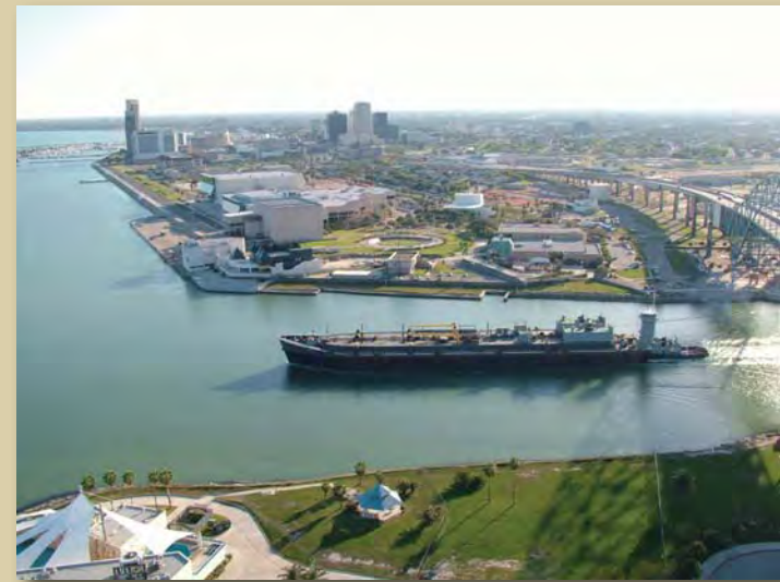
Port of Corpus Christi, TX. Credit: Port of Corpus Christi Authority
