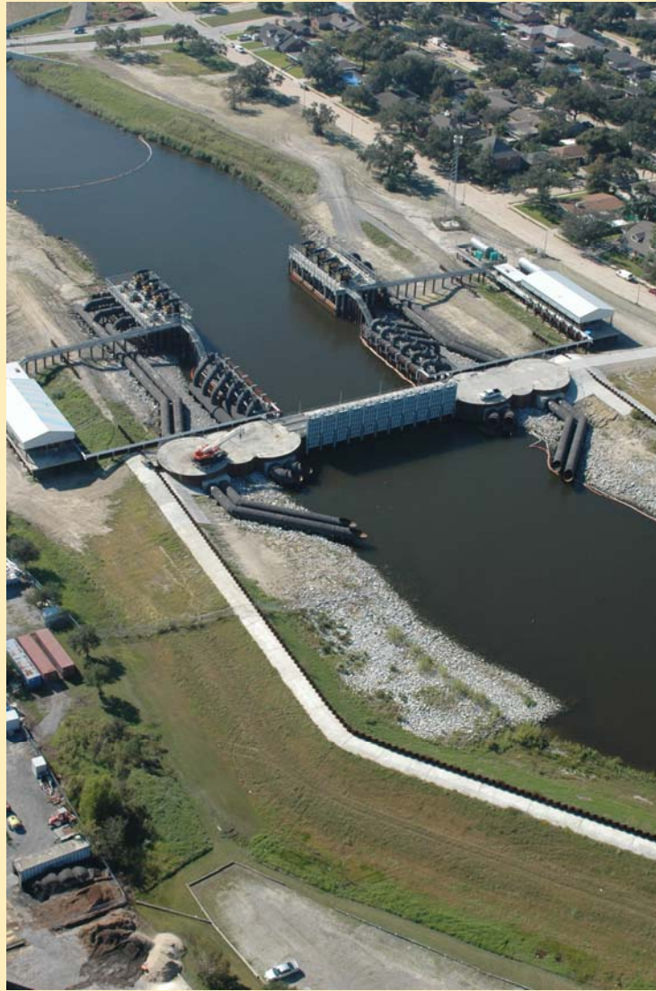
London Ave. Outfall Canal Interim Closure Structure
