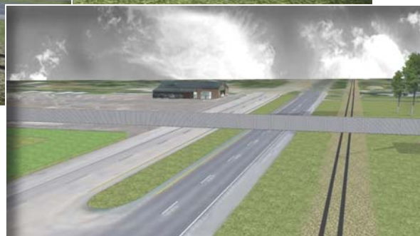
Finally, aluminum floodwall sections complete the closure of the system across Hwy. 23.
