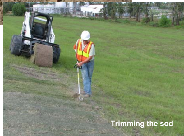
HPTRM with soil, and sod being added
